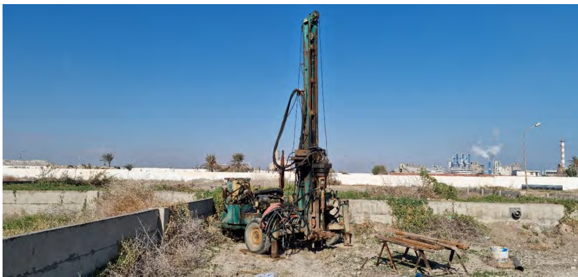
Figure Drilling Rig in BH 1
