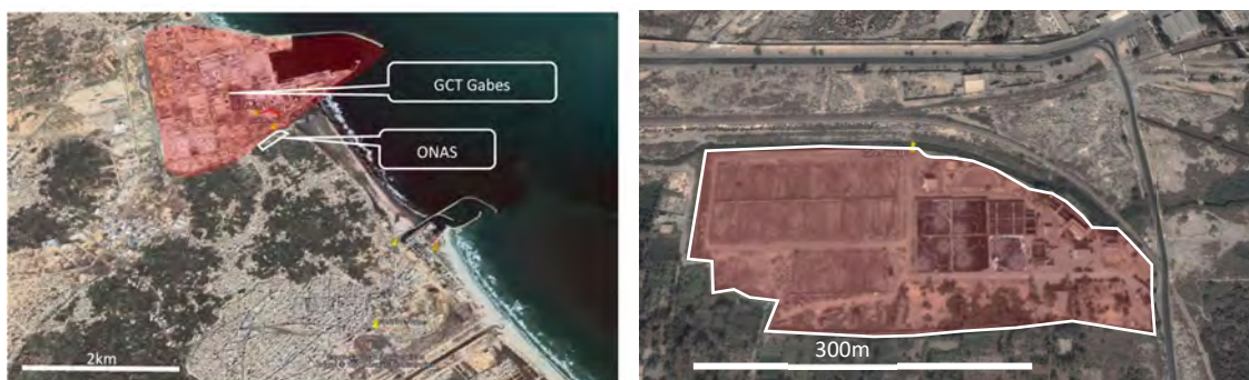
Gabes wastewater treatment plant and GCT Gabes Plant
