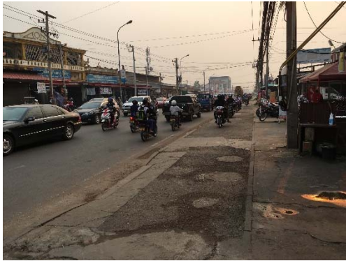
Figure 11.3-14 Unclear Road Markings
