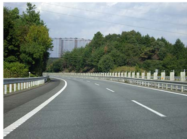
Figure 12.2-15 Properly Maintained Road
