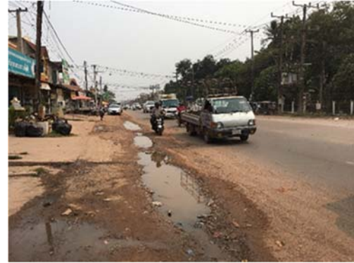
Figure 11.3-15 Insufficient Road Drainage
