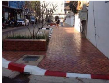
Improvement of sidewalk and parking space (Vientiane)
