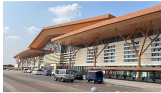
Figure 2.2-3 Lao-China Railway (Vientiane Station)
