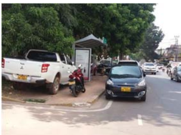
Illegal Roadside Parking
