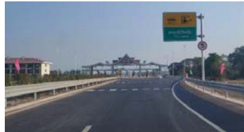
Vientiane-Vang Vieng Expressway
