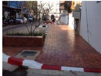
Improvement of sidewalk and parking space (Vientiane)
