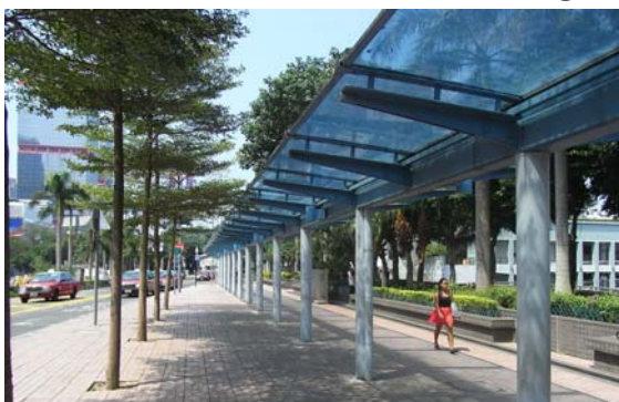
Wide Sidewalk with Sheds and Trees
