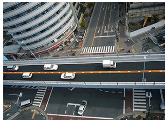
Flyover in Tokyo Source: Tokyo Metropolitan Government HP
