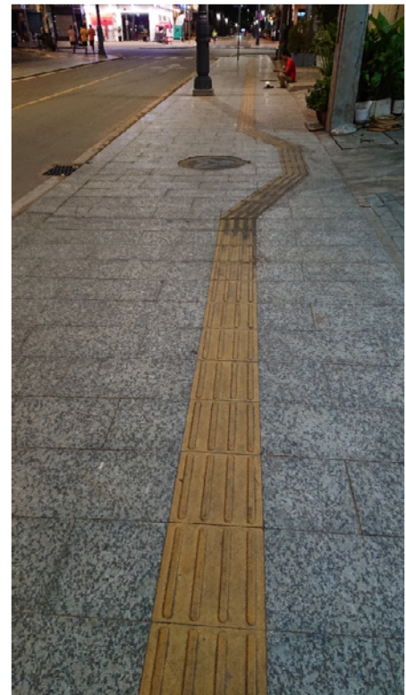
Wide Sidewalk with Blind guidance blocks in Siem Reap, Cambodia
