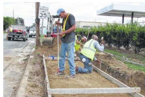
Sidewalk construction
