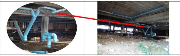
As a countermeasure to the clogging of the drainage pipe of the high-floor ward, the piping is cut off and the drainage water flows directly to the ground.
