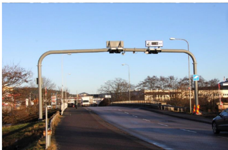
Figure 2.3.2 Example of Fixed ANPR Gantry in Gothenburg
