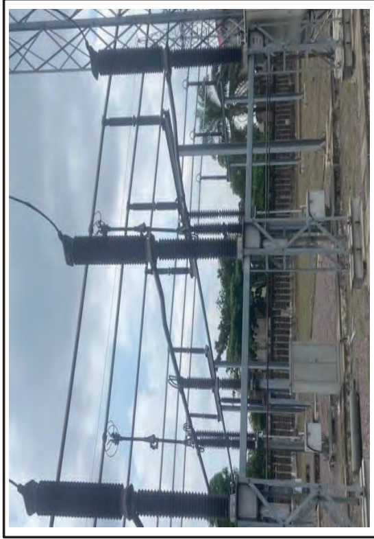
Photo n° 03 : La Funa substation surge arrester
