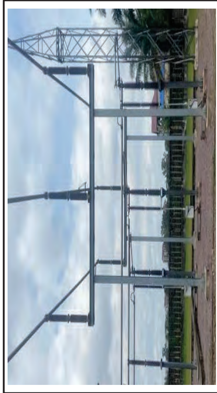
Photo n°07 : La Funa substation neutral point disconnector
