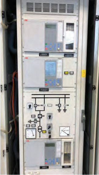
⑤ Armoires commande/control/protection , FUNA (exemple)
