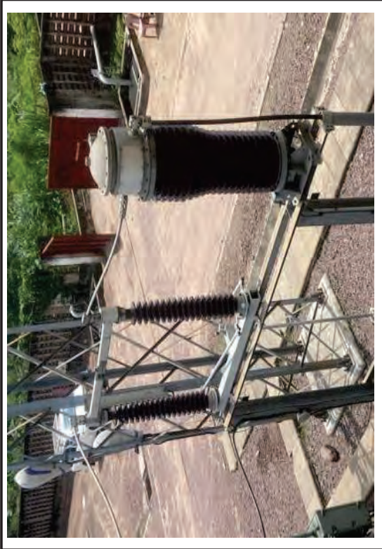
Photo n°07 : La Funa substation neutral point disconnector
