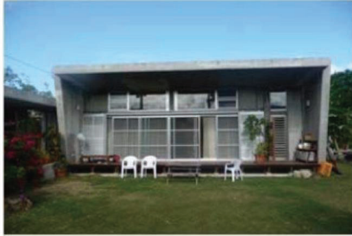
Windows at high position (from outside)
