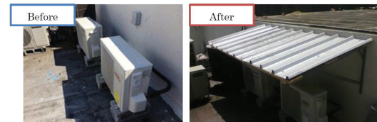
Construction of heat shielding
