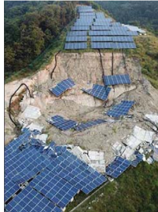
26 Jul 2019 Himeji, Japan https://www.dailyshincho.jp/article/2018/07/26/0800/?photo=1 Landslide by a heavy rain
