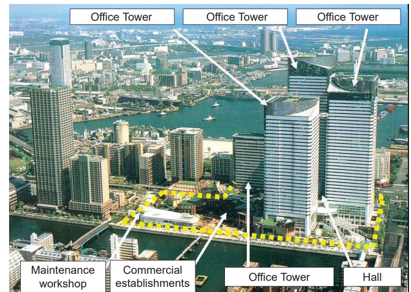
Harumi Island District Heating & Cooling, DHC
