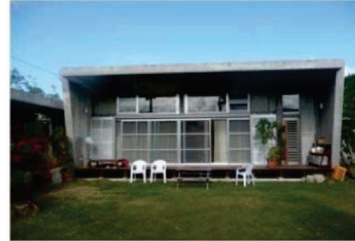
Windows at high position (from outside)
