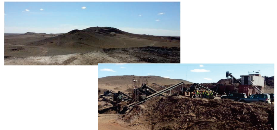
Complete view of the existing crushing plant
