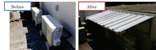
Construction of heat shielding
