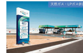
@ Liquefied petroleum gas station
