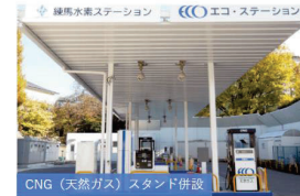
@ Compressed Natural gas station
