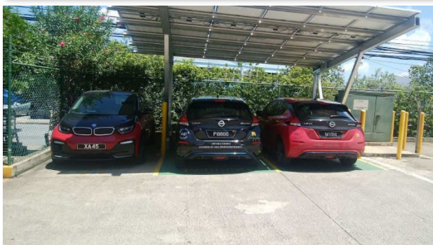
Photographs: Wind Farm in Jamaica / EE Testing Laboratory in Jamaica Solar PV System in St. Christopher Nevis / Coverley Village in Barbados EVs and Quick Charging Spot with Solar PV in Barbados
