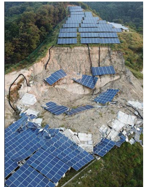
26 Jul 2019 Himeji, Japan https://www.dailyshincho.jp/article/2018/07260800/?photo=1 Landslide by a heavy rain
