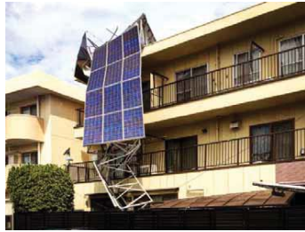
9 Sep 2019 Kanto, Japan @kadowaki_kozo Damage of roof-top structure by high speed wind
