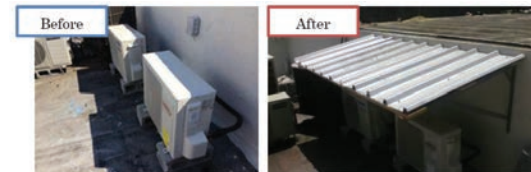
Construction of heat shielding
