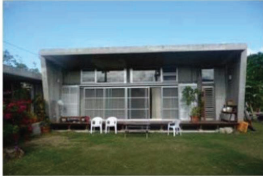
Windows at high position (from outside)
