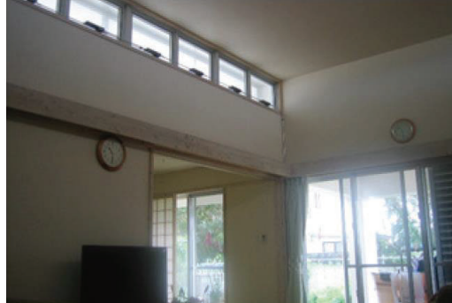
Windows at high position (from inside)
