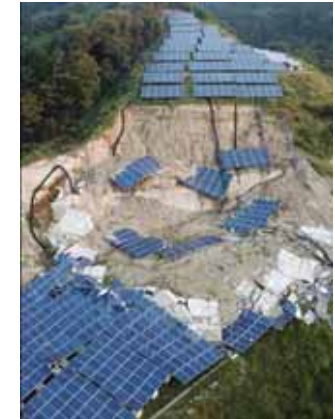
26 Jul 2019 Himeji, Japan https://www.dailyshincho.jp/article/2018/0726/0800/?photo=1 Landslide by a heavy rain
