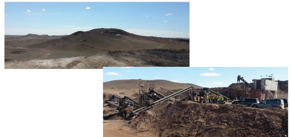
Complete view of the existing crushing plant
