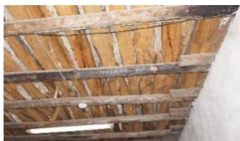
Figure 56: Structure of the Floor (viewed from behind the floor)
