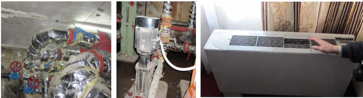
Figure 17: Hotel hot water receiving system, pressure booster pumps, and fan coil unit
