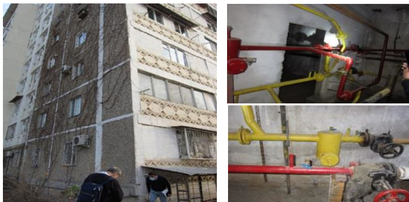
Figure 22: Hot water piping and return water piping for the heat receiving system in the basement floor of a 9-story apartment building
