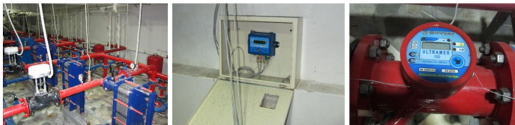
Figure 16: Closed system hot water receiving facilities, calorimetric metering equipment, and calorimeters at elementary and junior high schools
