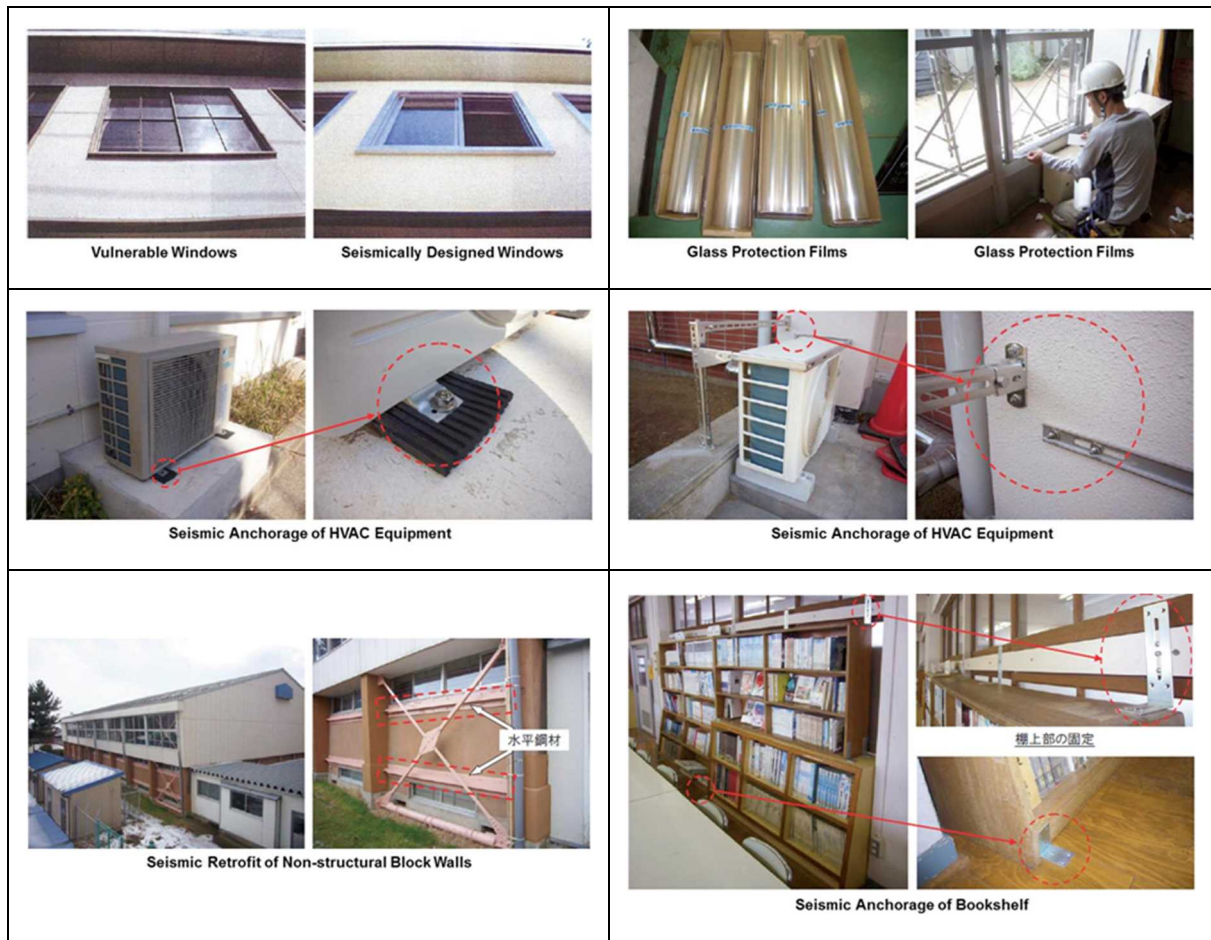
Source: Case studies of seismic countermeasures for nonstructural components of school facilities (Ministry of Education, Culture, Sports, Science and Technology).
