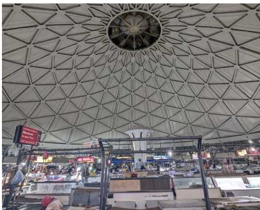
Chorsu Bazaar A distinctive building with a latticed dome that achieves a large space without pillars
