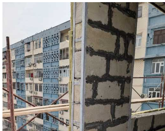
A material, foamed concrete, commonly used for walls in modern reinforced concrete buildings. It has good insulation and, when dry, matches brick strength but is less dense. Joints are filled with cement and reinforced horizontally, but not vertically.
