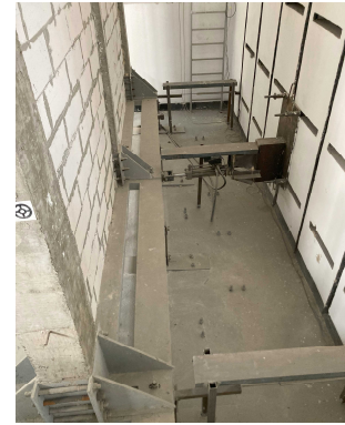
Experiment on reinforcement of brick walls with Basalt
