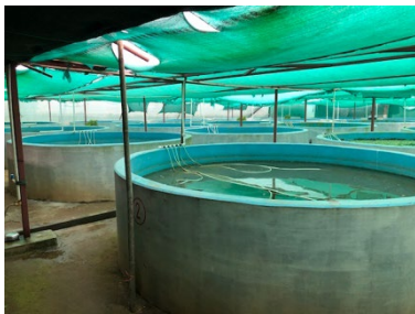
Circular concrete tank with biofloc system
