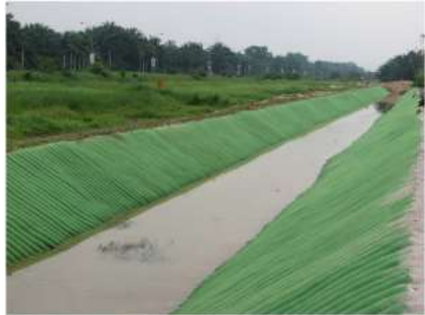
写真 3.6.7 Sand Filled Mattress
