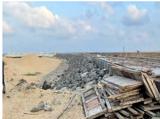
Right bank Training Wall
