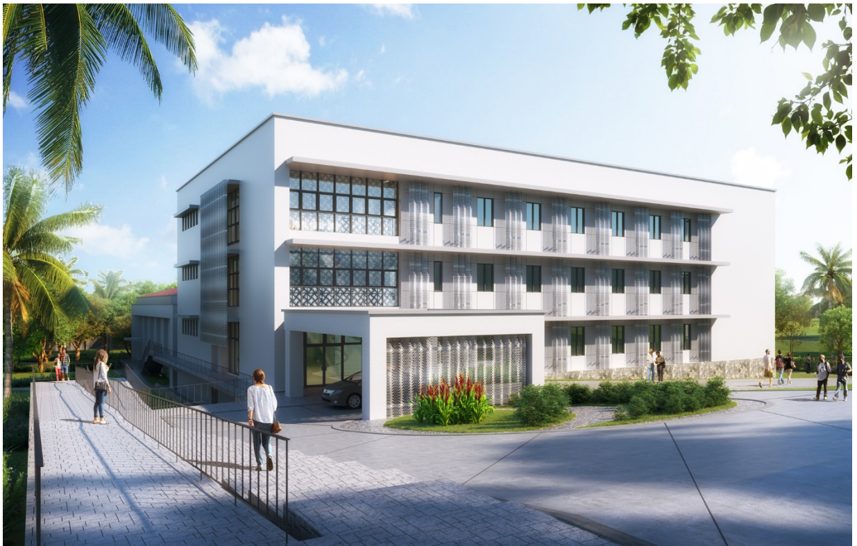
Figure IV South Side View
