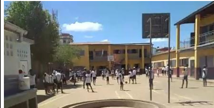
Junior high school, separate toilets for girls and boys on the left, separate gym for girls and boys.
