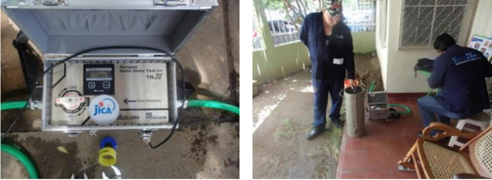
Figure 2.9.1 Example of a test meter and a standard tank
