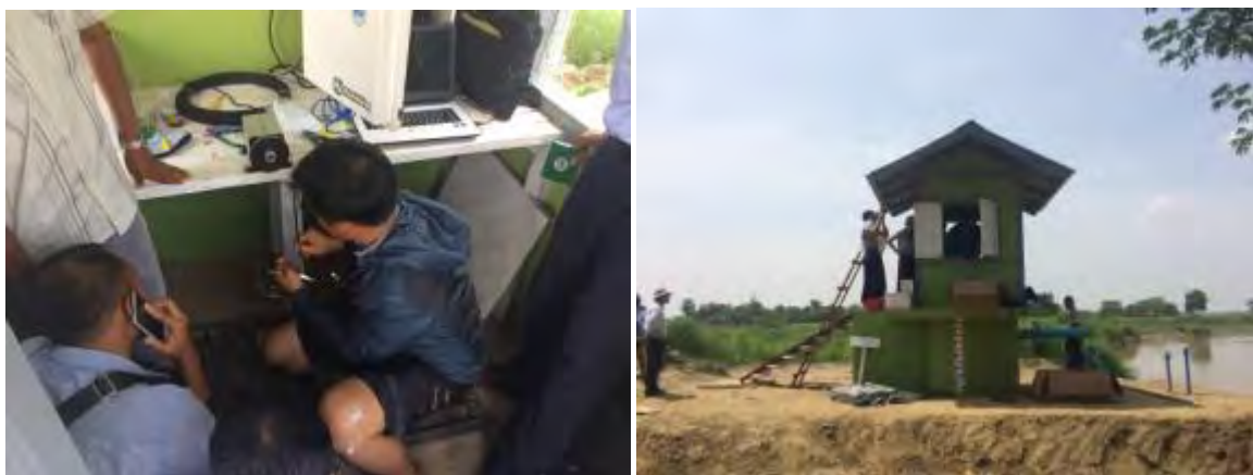
Fig.2 Installation of water level station at Tawa sluice gate .
