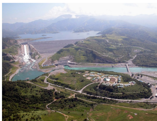
Figure 3.5-1 San Roque Dam and Hydropower Plant
