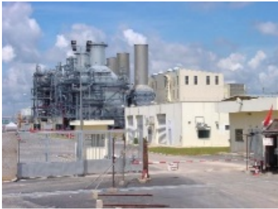
Figure 3.5-3 Phu My 1 Power Plant
