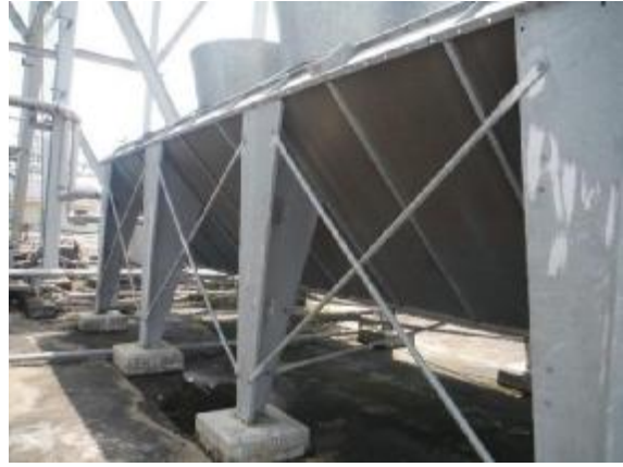
Gas Turbine Common Issue No.2
