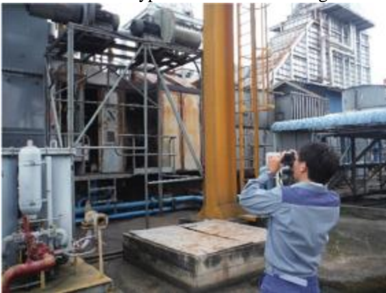
Leakage Diagnosis by Thermal Camera
