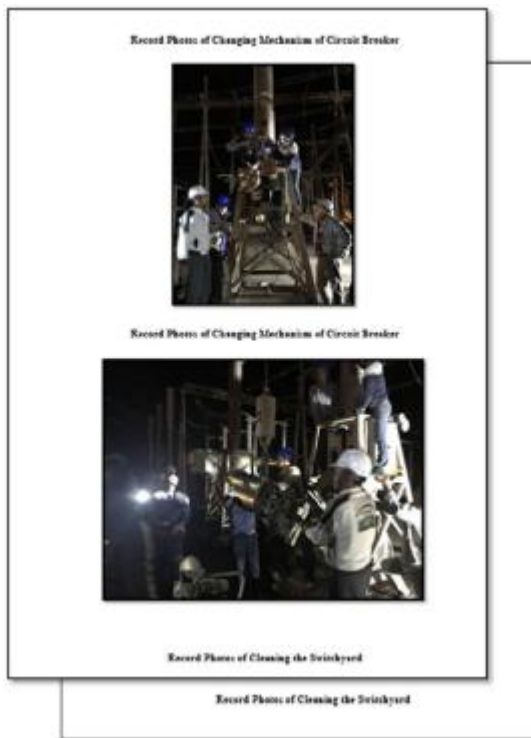
Fig. Record of CB Replacement Work
