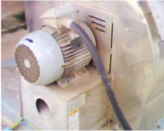
#2 GT Motor of Lube Oil Mist Separator Fan
