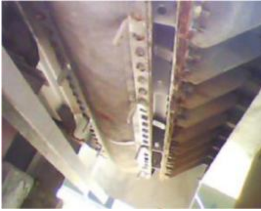
#2 GT Chimney Inlet Expansion
