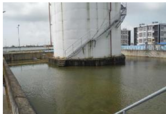
Fuel Tank Yard Storing Rain Water
