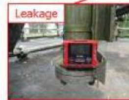
Strainer level gauge lower side flange (100%LEL)
