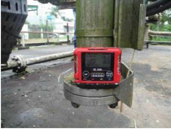
Strainer Level Gauge Flange Gas Leakage
