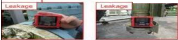
Dangerous operation in gas leakage condition
