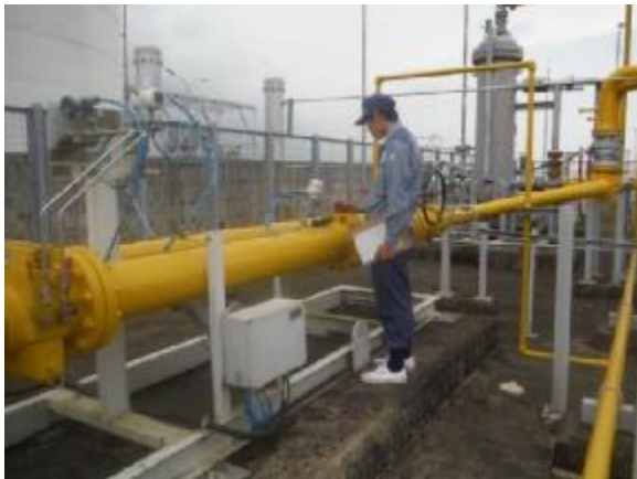
Gas Leakage Check
