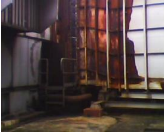
GT Exhaust Duct Overheating (#1, 2, 3 GT)
