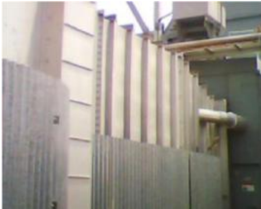
#2 GT Exhaust Gas Duct
