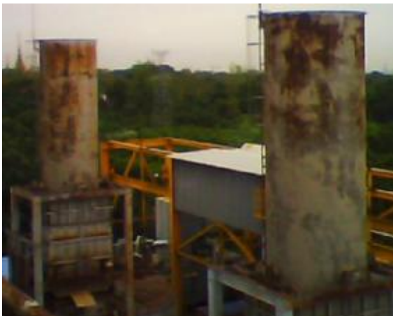
HRSG Bypass Stack Overheating due to Damper Gas leakage (#1HRSG, #2HRSG)
