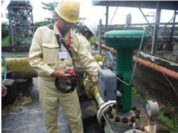
Gas Leakage Check
