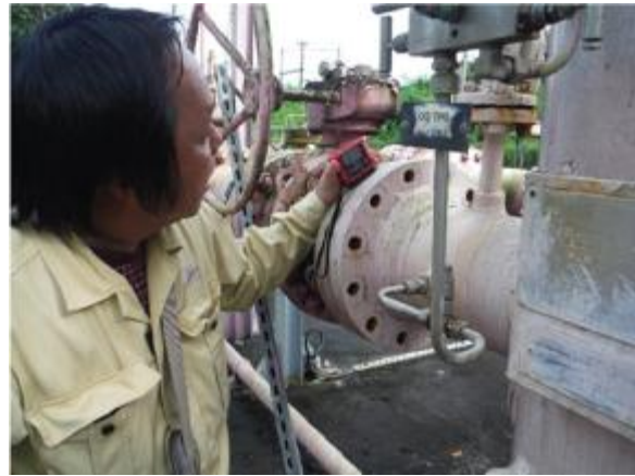
Gas Leakage Check
