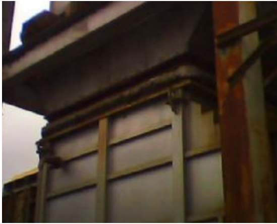
Bypass Stack Expansion Joint Gas Leakage (#1, 2, 3 HRSG)
