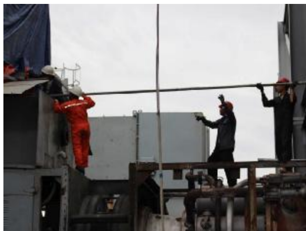
Fig. Periodic Inspection Execution Scene
