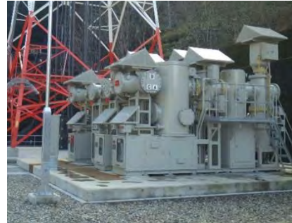
図 5-21 GIS(Gas Insulated Switchgear)
