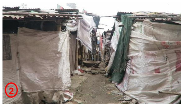
They cover their structures with plastic sheets.
