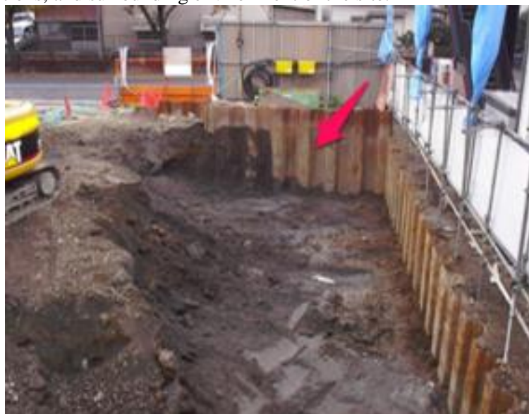
Figure 14-23 Explanation of Steel Sheet Piling
