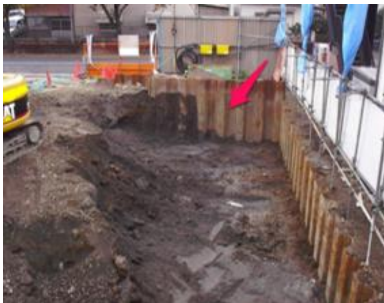
Figure 6-24 Explanation of Steel Sheet Piling
