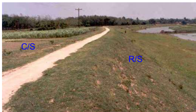
Figure-1 Flood Management Embankment
