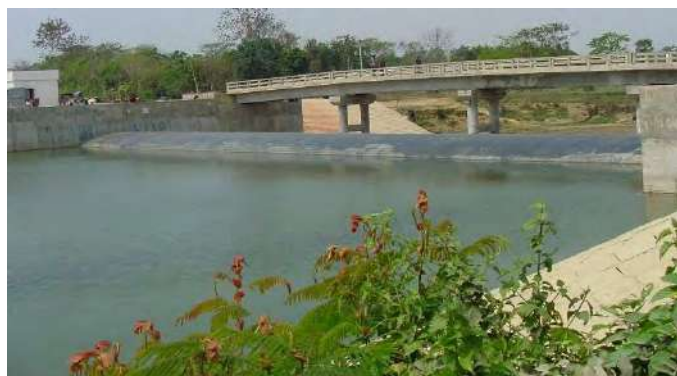
Figure-11 Rubber Dam
