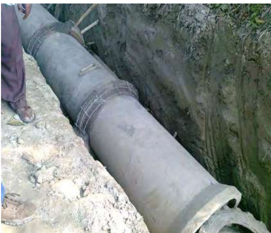
Placement of concrete surround to joints with concrete mortar / bitumen in the joints
