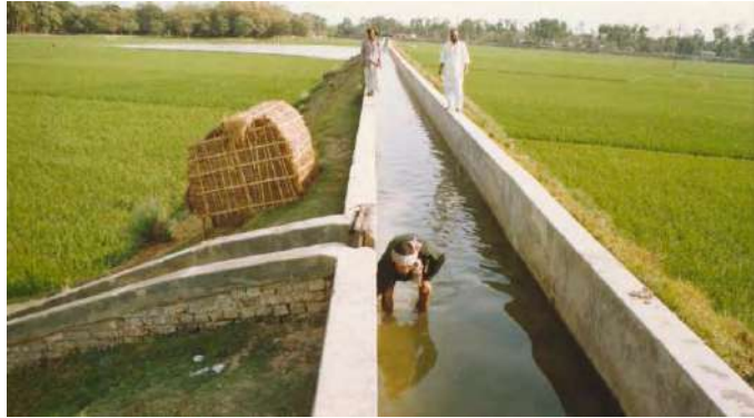
Figure-7 Irrigation Canal
