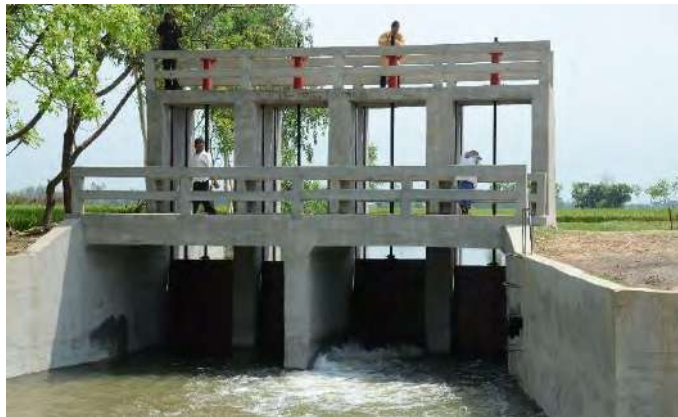
Figure-5 Water Conservation Structure
