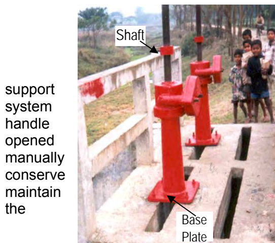
Figure-13 Raising of Vertical Gate
