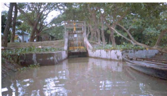
Figure-15 Flap gate lifting system
