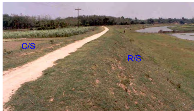
Figure-1 Flood Management Embankment
