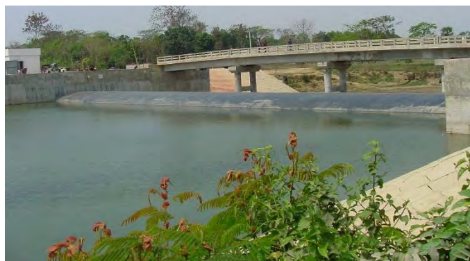
Figure-11 Rubber Dam
