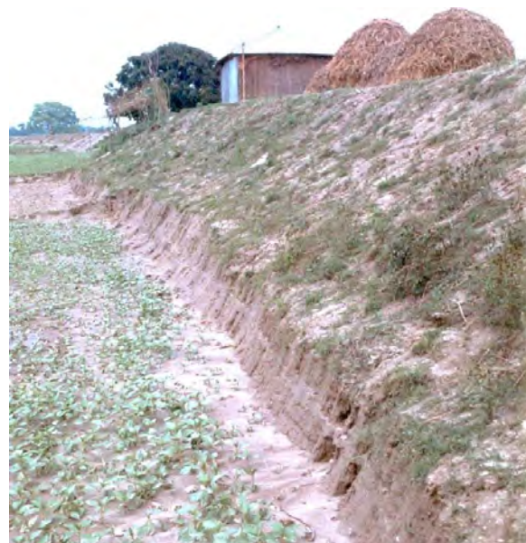
Figure-22 Cutting of Toe of Embankment
