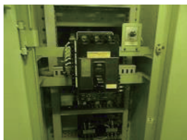
Circuit breaker of switch board (Caroline Voyager)
