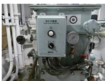
Oil separator (Micronesian Navigator)
