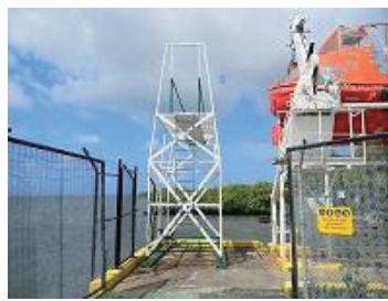
Lifeboat waiting for repair and platform for jumping without sufficient depth of water
