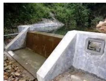
Figure 7.9: Spring Tapped Chamber
