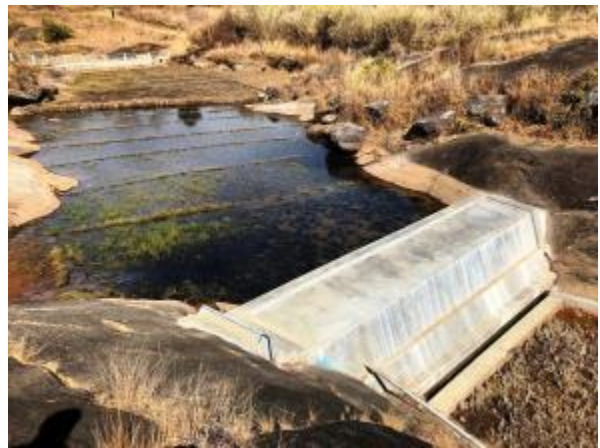
Utilization of eroded soil and spring water collected by check dam as paddy field in Mawshut Village, West Khasi Hills District
