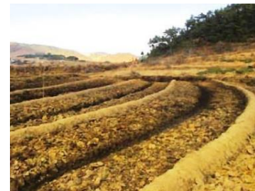
Figure 7.4: Earthen/Loose Boulder Contour Bund
