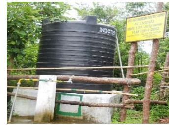
Figure 7.12: Drinking Water Tank
