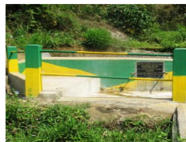
Figure 7.8: RCC Water Storage Tank for Drinking Water
