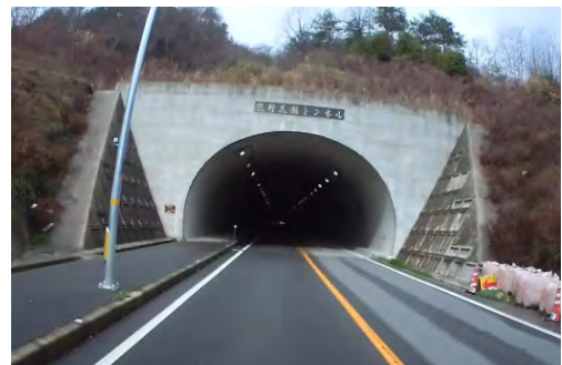
Figure 2.10 Kumano Hirose Tunnel
