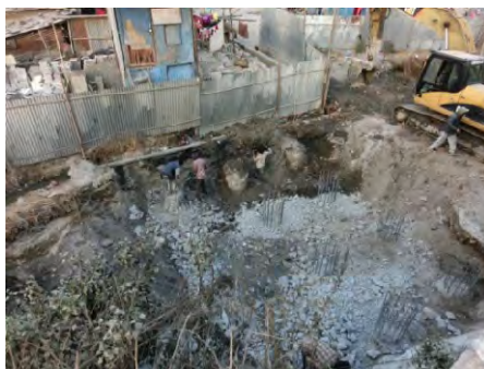
Figure 4.5.2 Photo of the Construction of Cast-in-Situ Concrete Pile in Kathmandu
