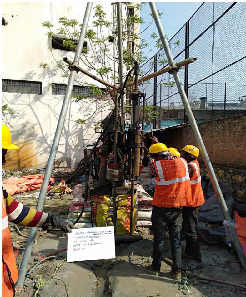
Conducting SPT/DCPT Test for getting (N) Value by Dropping 63.5 kg Hammer from 750mm height
