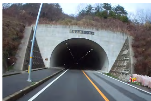
Figure 2.10 Kumano Hirose Tunnel
