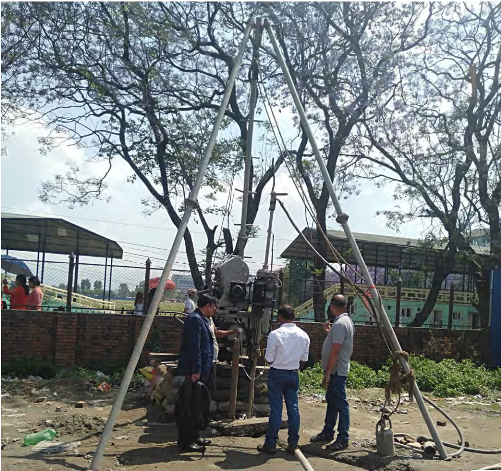
Conducting Methane Gas Test
