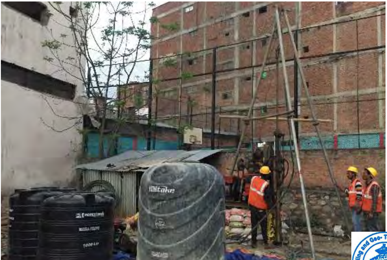
Drilling a Hole by Rotary Drilling Method
