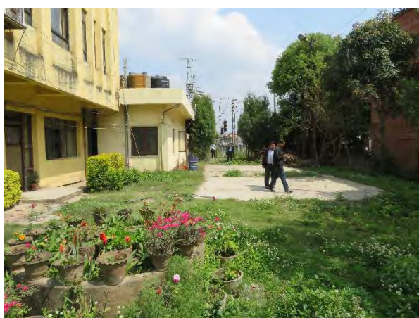
Figure 4.3-9 Baneswar substation compound
