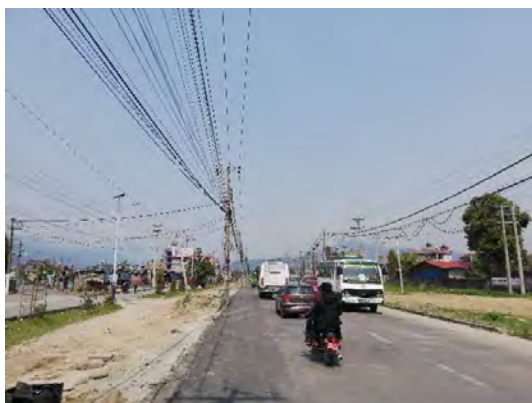
Figure 4.2-11 Congestion of distribution feeder on the west side
