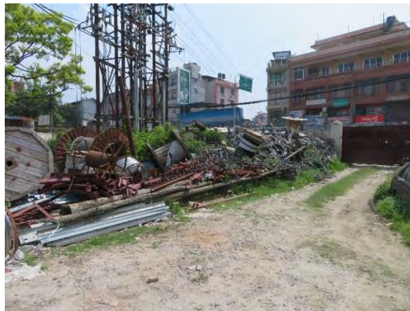
Figure 4.3-8 Compound of Maharajgunj switching station
