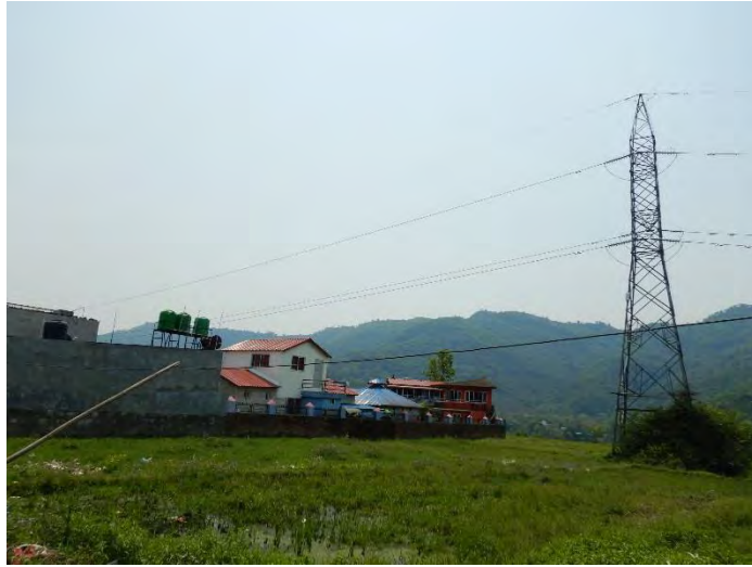
Figure 4.2-7 Picture of existing tower for junction
