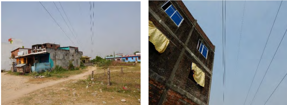
Figure 4.2-25 Situation under the existing transmission line between Kohalpur and Bhurigaon
