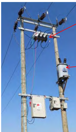
Control source Transformer 22/0.2kV
