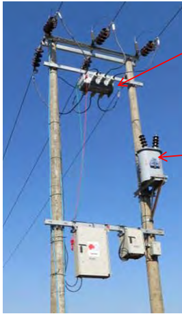
Control source Transformer 22/0.2kV
