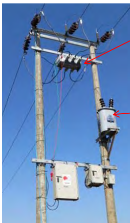
Control source Transformer 22/0.2kV
