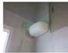
Light insect trap shall be equipped so that light cannot be seen from outside, other wise it attract insect from outside.
