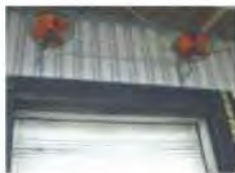
Wind from fan to prevent insect entrance
