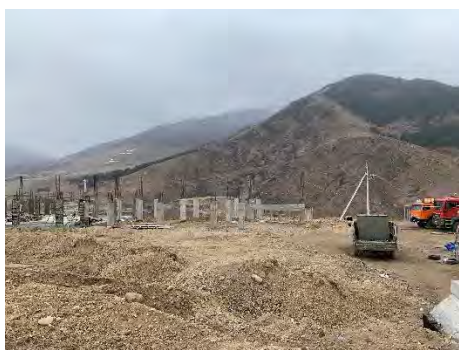
Construction site of RSS
