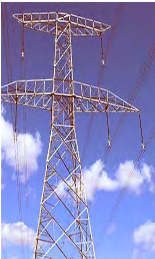
Figure 8.8.7 Example of 220-kV Double Circuit Lattice Steel Tower
