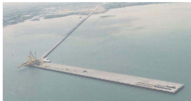
Figure 8.3.16 Offshore Container Terminal with Access Bridge of Tanjung Perak Port
