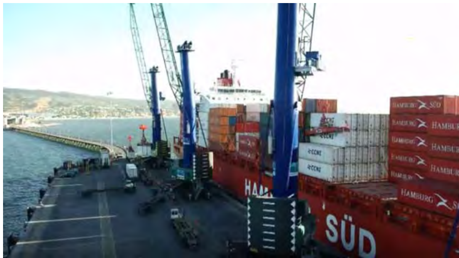
Figure 8.3.53 Tractor-chassis Turning on the Jetty (Jetty width: about 50m)
