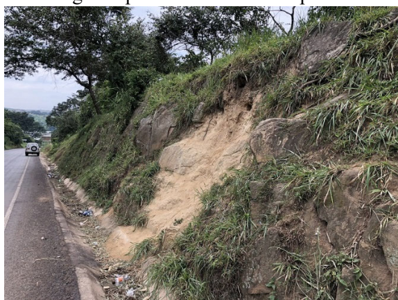
Rock cut on Gulu side approach road (the right bank)
