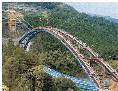
Construction of Steel Arch using Temporary Cable Crane
