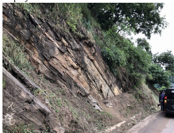
Rock cut on Kampala side approach road (the left bank)
