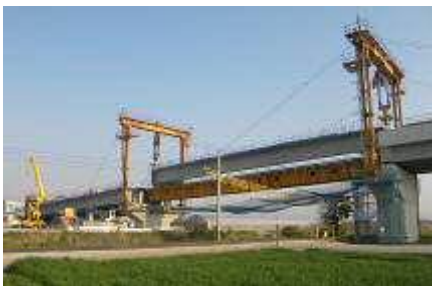
Figure 3.4.5. Erection Girder Construction Method for Prestressed Concrete Girder
