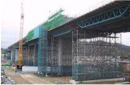
Figure 3.4.4 Temporary Support Method for Concrete Bridges
