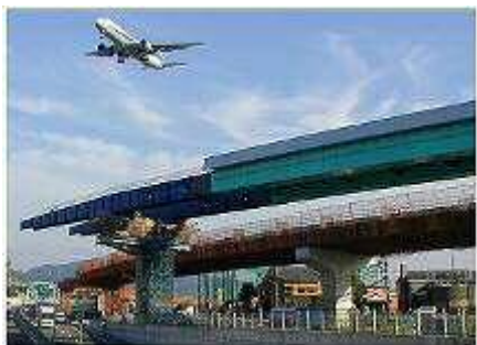
Figure 3.4.6 Incremental Launching Method of Steel Girders
