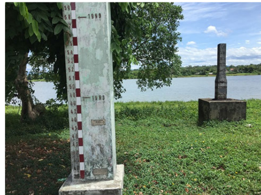
No-dike section (middle stream, urban area)
