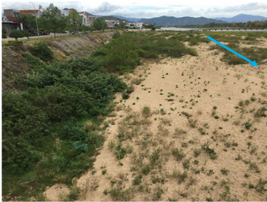
No-dike section (middle part)
