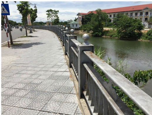
No-dike section (middle stream, urban area)
