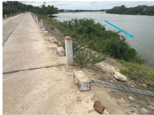
Dike section (downstream)
