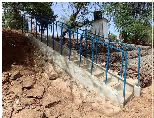
Completed stairs with hand rail and river bank protection (4F10, 2019/03/01)
