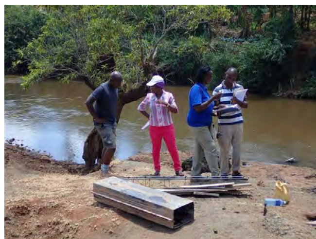
Steel form and reinforcement bars for construction of a concrete post to fix staff gauge (4BE10, 2018/02/22)
