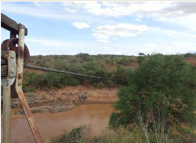
Crossing cable for moving a cage (4F13, 2017/06/14) (No usage for long time)
