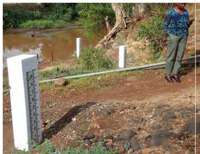
Completed staff gauge posts (4DD02, 2019/03/02)
