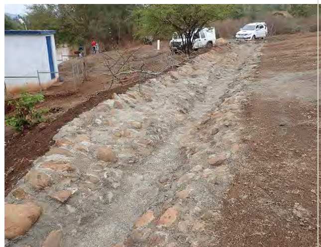
Completed drain canal (4BE10, 2019/03/02)
