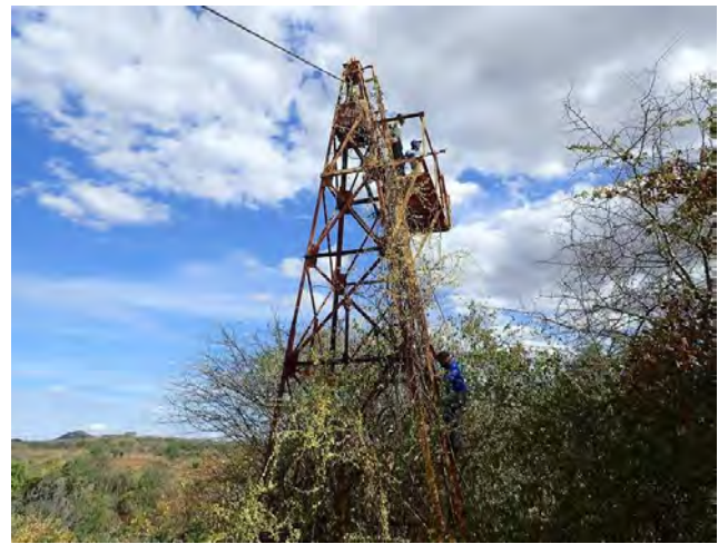
A tower to stay cables for discharge measurement (4F13, 2017/06/14)
