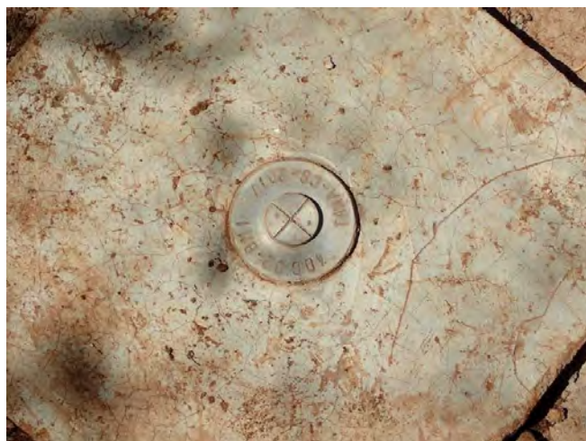
Bench mark for river cross section survey (4DD02, 2017/10/12)
