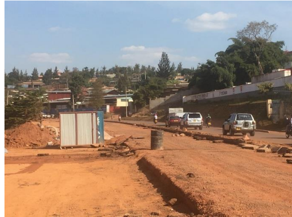
On-going widening to 4-lane at KN3 Road
