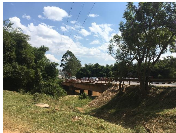
Existing Bridge on Nyabarongo River (2-lane)
