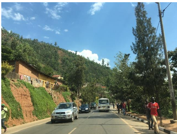
Existing Condition (2-lane and shoulders with no sidewalk), Pavement is in Good Condition
