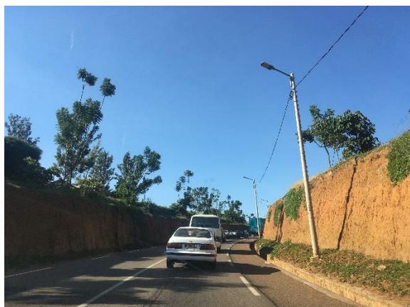
Existing Condition of NR5 (2-lane)
