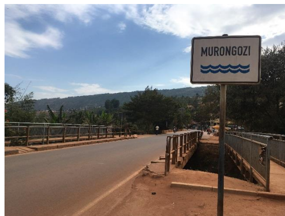
Existing Bridge on Murongozi River (2-lane)
