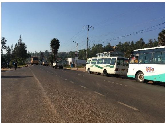
Two Lanes, Good Condition of Pavement
