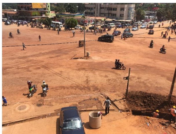
Current Situation of Nyabugogo Intersection: Under Construction
