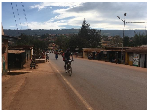
Existing Condition (2-lane)
