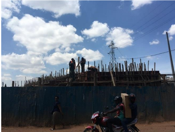
Nyabugogo Bridge under Construction
