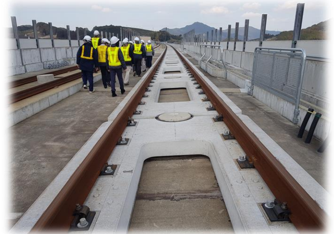
Track laid on Slab
