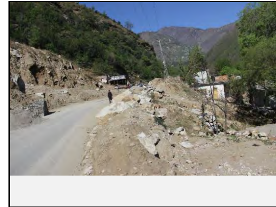
Front view of the debris flow
