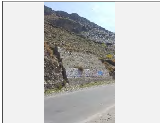
Existing countermeasures / anomalies: View of Stepped Retaining Wall as counter measure
