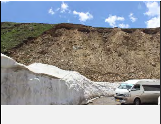
The new slope failures has been found along the debris flow
