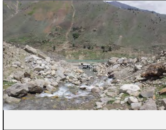
Valley side view of the debris flow
