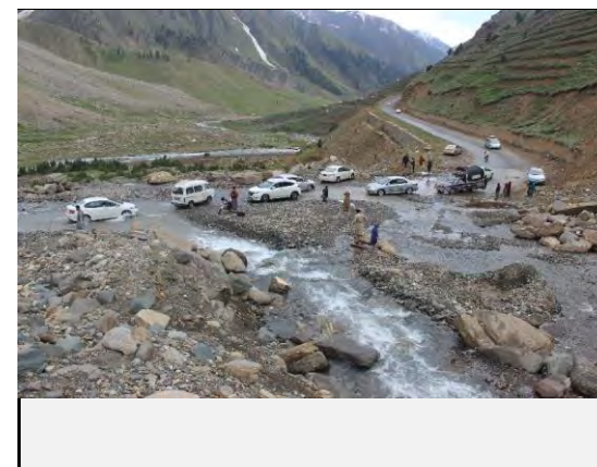
Debris flowing on road
