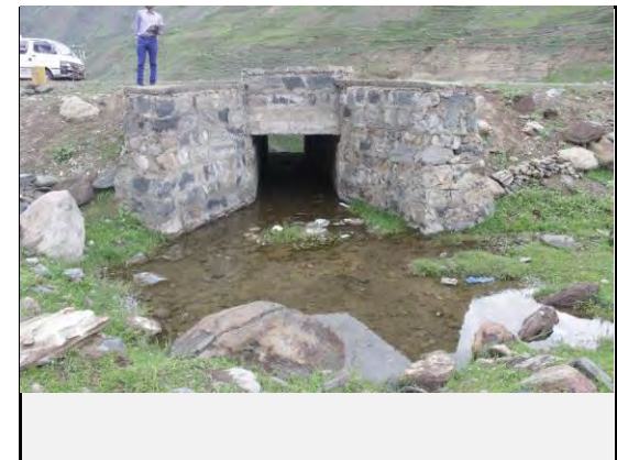
View of Box Culvert at the toe of slope
