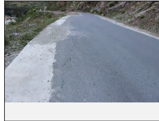
Road condition: Cut slope at the start point
