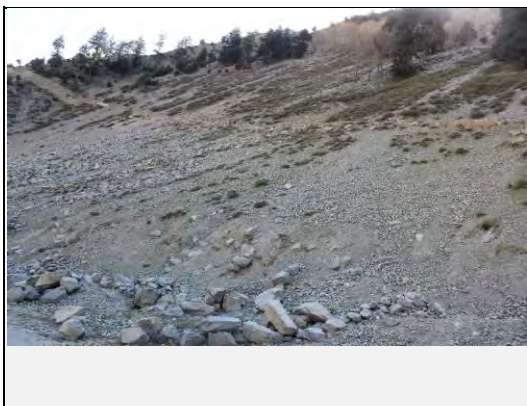
Full view of the slope failure
