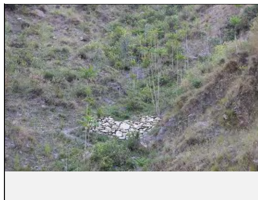
Existing countermeasures / anomalies: View of check dam as counter measure
