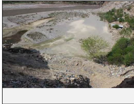
View of landslide on Valley side:
