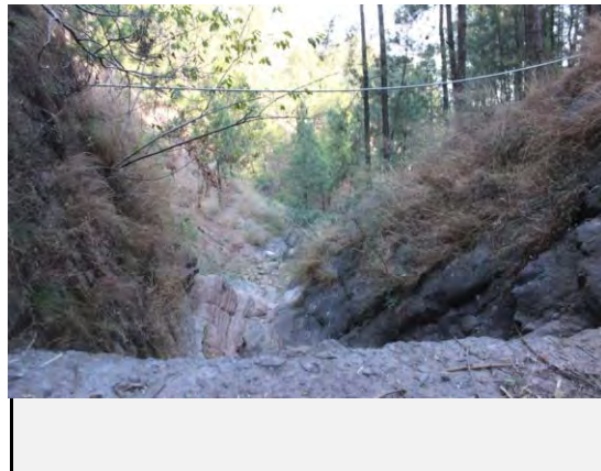
Valley side view of the debris flow
