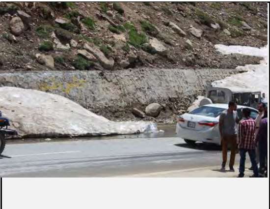
Existing countermeasures / anomalies: Retaining wall has been constructed along the Debris Flow
