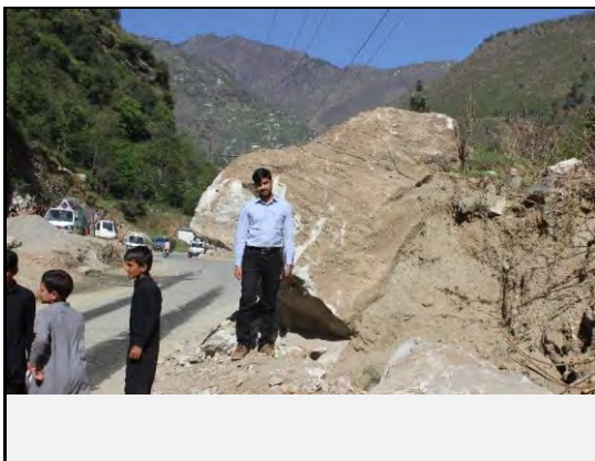
View of fallen block with the debris flow that can damage the population along the downstream.
