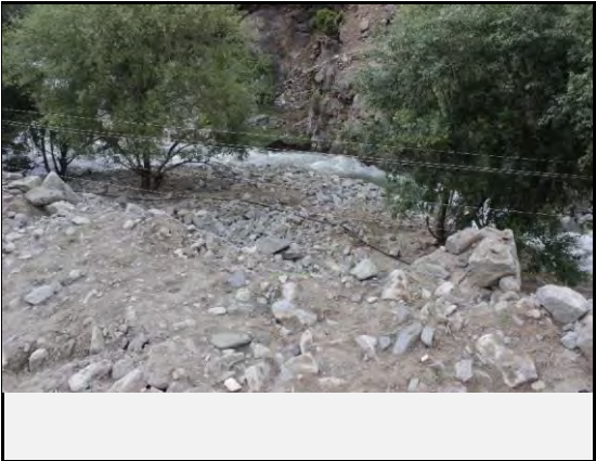
Valley side view of the debris flow
