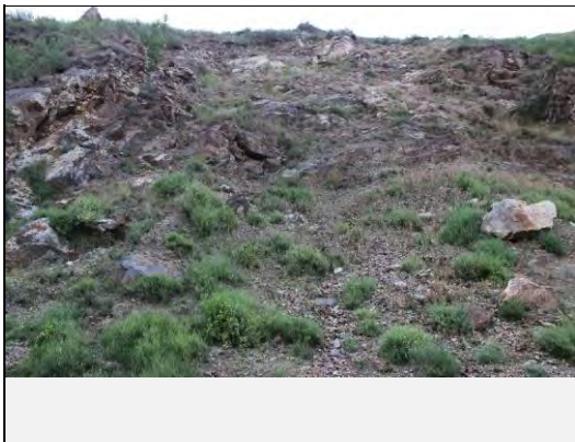
View of the slope failure at the middle point
