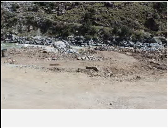
Valley side view of the debris flow
