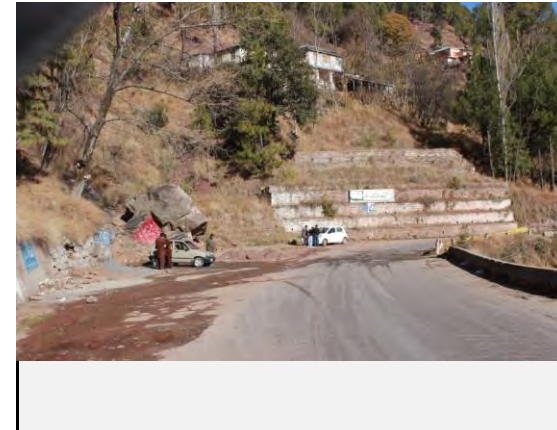
Road condition at location
