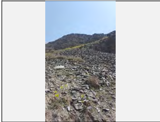
Full view of the slope failure
