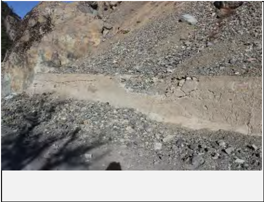
Existing countermeasures / anomalies: View of Retaining Wall as counter measure
