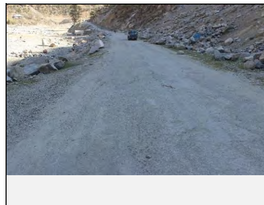
Road condition: Cut slope at the start point
