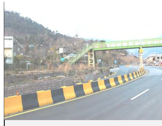
Road condition: Road passing through the center of the landslide
