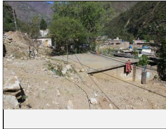
Valley side view of the debris flow
