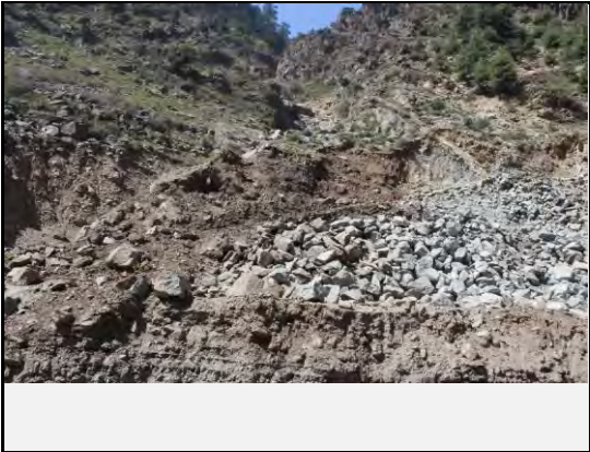
Front view of the debris flow
