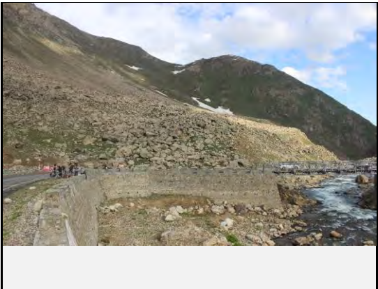
View of the toe of Landslide cut by the stream
