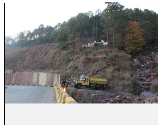
Existing countermeasures / anomalies: Retaining wall has been constructed at the toe of the slope failure
