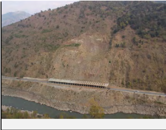
Full view of the landslide
