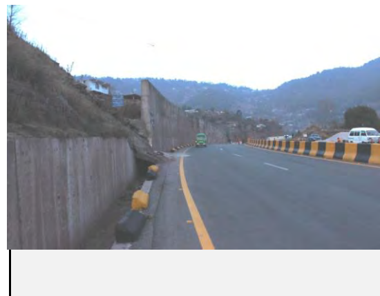
Existing countermeasures / anomalies: Retaining wall has been constructed
