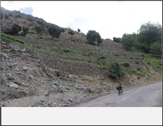
The Check dams has been built along the debris flow
