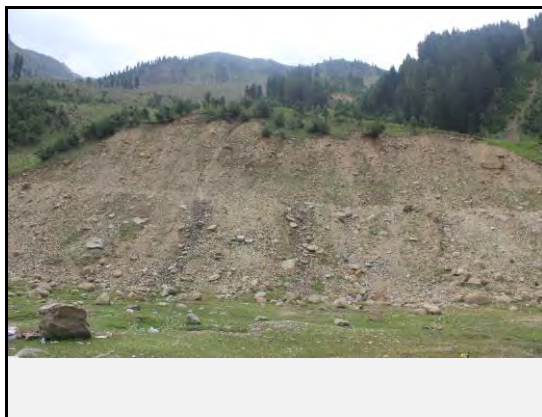
View of the Landslide at the middle point
