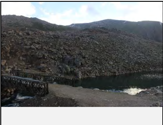
View of landslide on Valley side:
