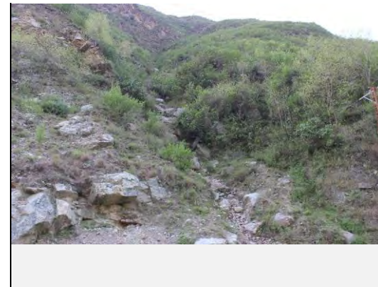
View of drainage that cuts the slope
