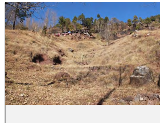
Construction of small check dams to control debris flow
