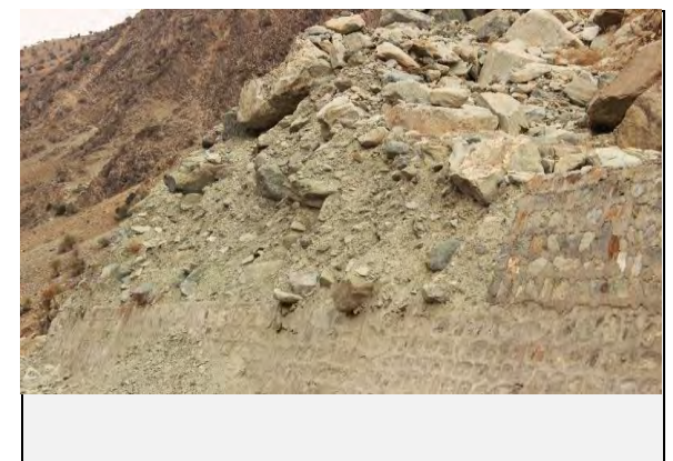
View of fallen blocks
