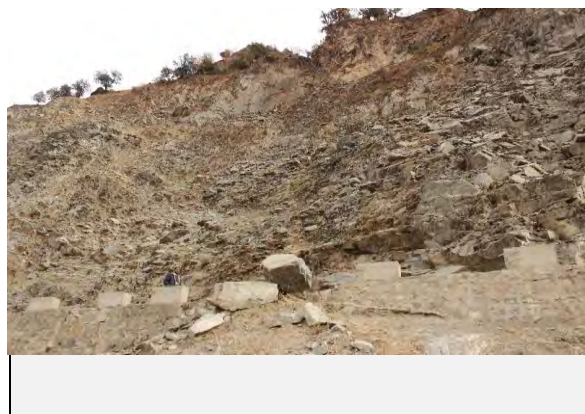
Full view of the landslide
