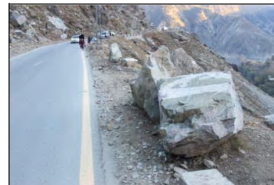
View of fallen blocks on road
