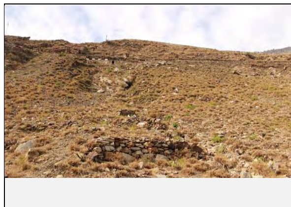
Full view of the landslide
