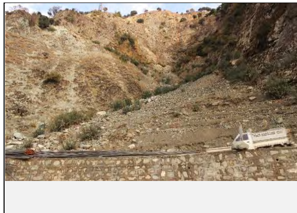
Existing countermeasures / anomalies: View of benching as counter measure
