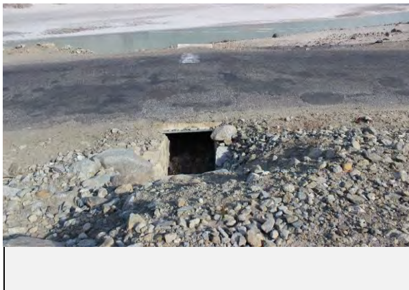
Inlet of the culvert for the debris flow
