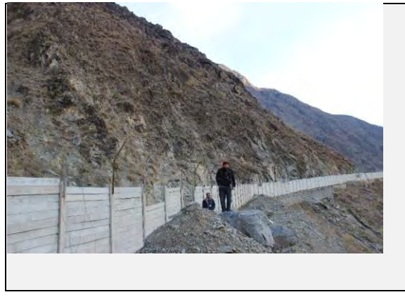
Existing countermeasures / anomalies: View of shed as counter measure
