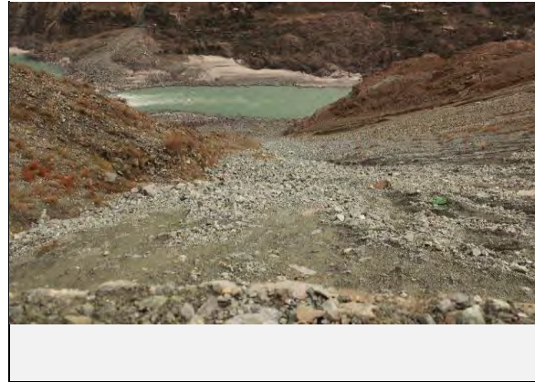
View of landslide on Valley side:
