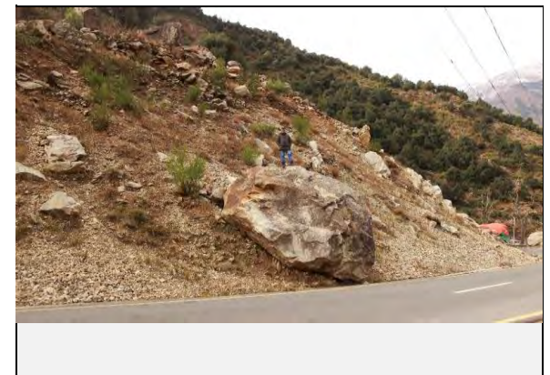
View of fallen blocks on road
