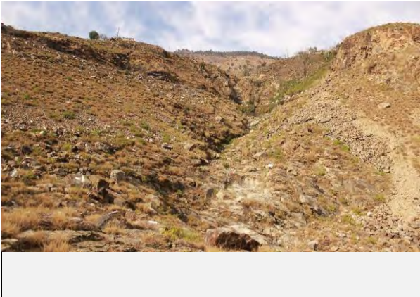
Valley side view of the debris flow
