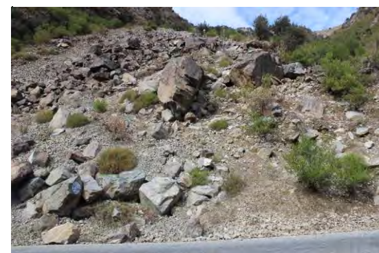
View of fallen blocks
