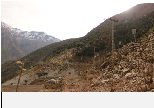
Full view of the landslide
