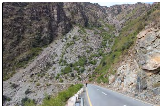
Full view of the landslide
