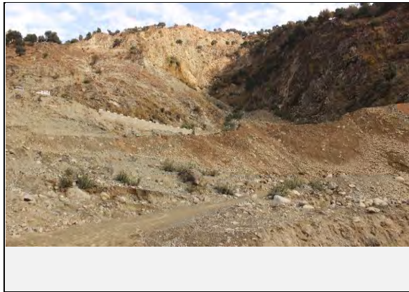
Full view of the landslide
