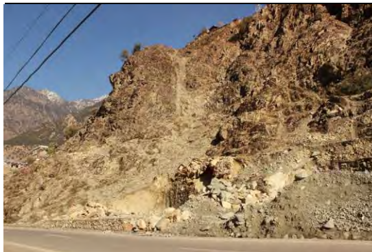
Existing countermeasures / anomalies: View of retaining wall as counter measure
