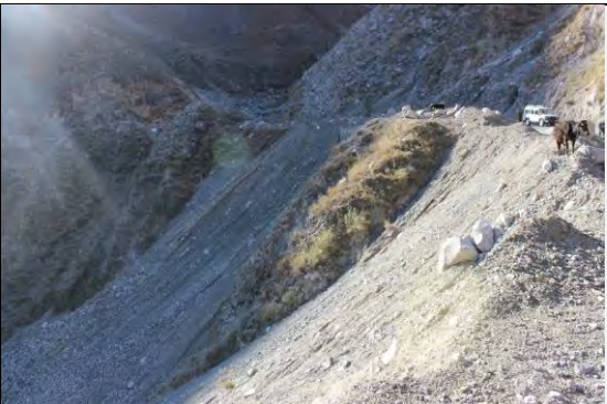
View of landslide on Valley side:
