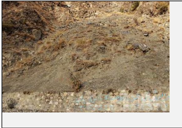
Full view of the landslide
