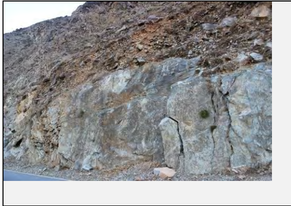
Full view of the landslide
