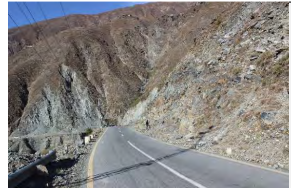
Road condition: Cut slope at the start point
