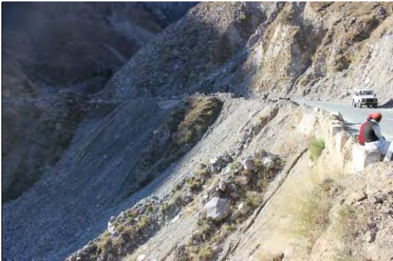
View of fallen blocks
