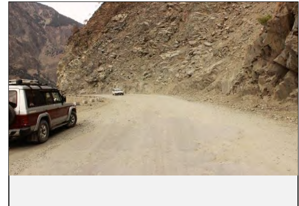
Road condition: Cut slope at the start point
