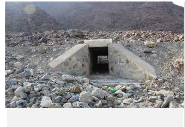
Existing countermeasures / anomalies: Culvert outlet view
