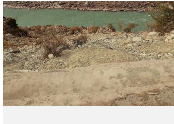
View of landslide on Valley side:
