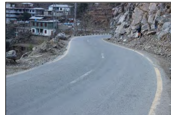
Road condition: Cut slope at the start point
