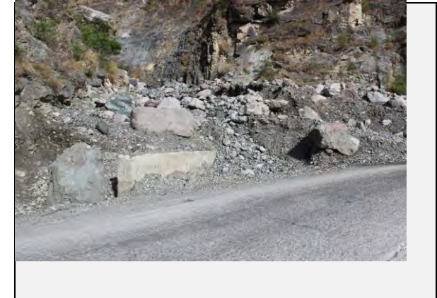
Front view of the debris flow
