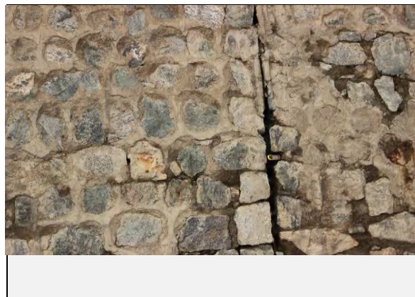
Existing countermeasures / anomalies: View of shed as counter measure
