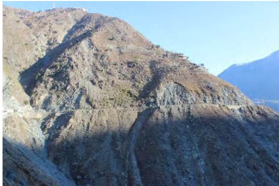
Full view of the landslide
