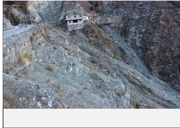
View of landslide on Valley side:
