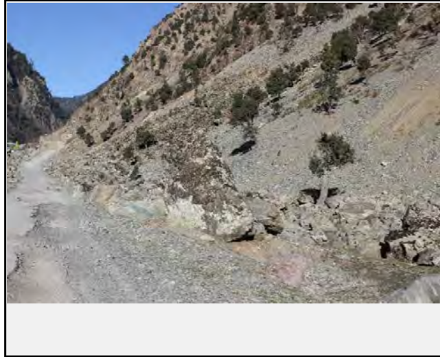
Full view of the landslide
