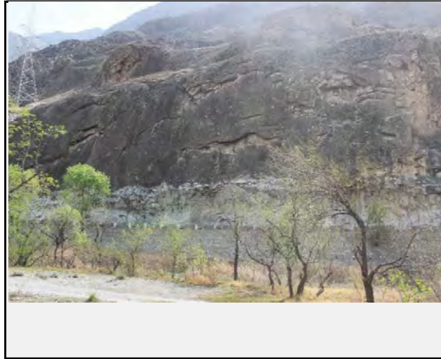
Full view of the landslide
