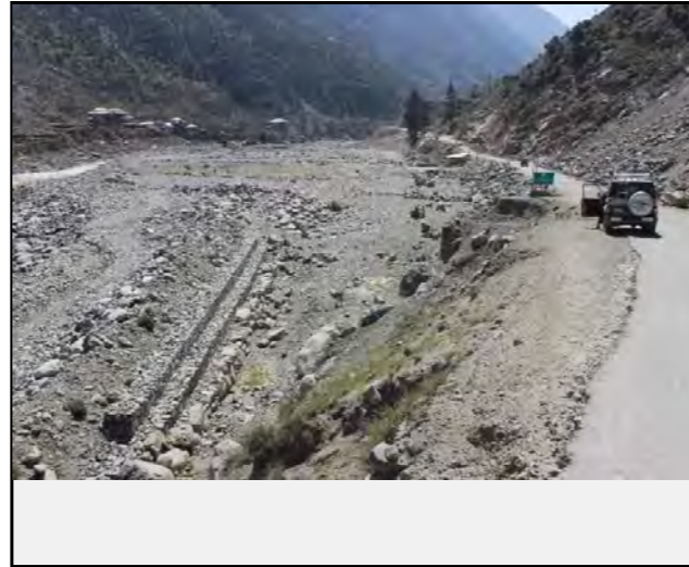
View of landslide on Valley side and a river diversion structure built on the toe of the slope failure
