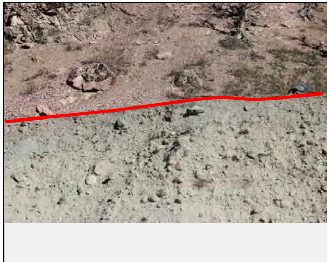
The existing road has been damaged. Red line shows the old road displaced by the debris flow.
