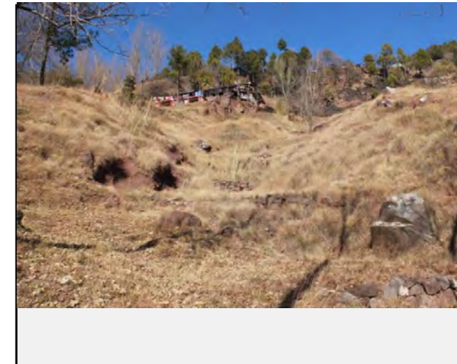
Construction of small check dam to control debris flow
