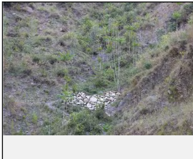
Existing countermeasures / anomalies: View of check dam as counter measure
