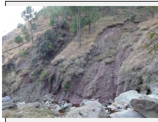
Existing countermeasures / anomalies: Several surface collapse can be observed on the west side of the slope on the mountain side.
