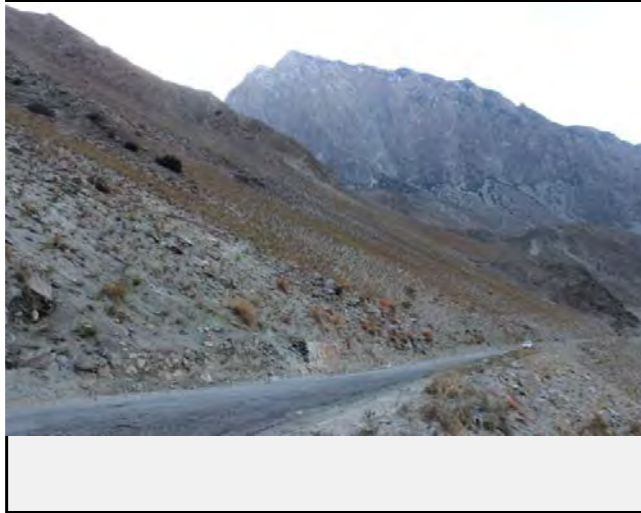
Full view of the landslide
