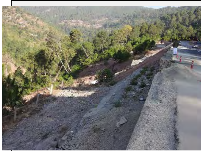
Existing countermeasures / anomalies: Surface erosion protection net are installed to minimize the surface erosion.
