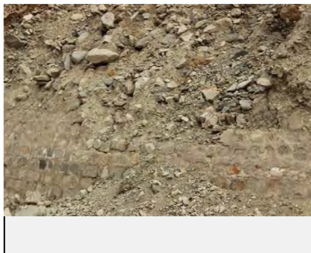
Existing countermeasures / anomalies: View of retaining wall as counter measure for slope failure
