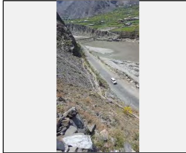
View of landslide on Valley side:
