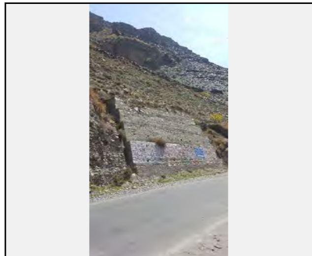
Existing countermeasures / anomalies: View of Stepped Retaining Wall as counter measure
