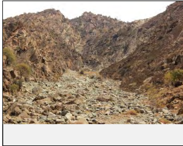
Full view of the slope failure
