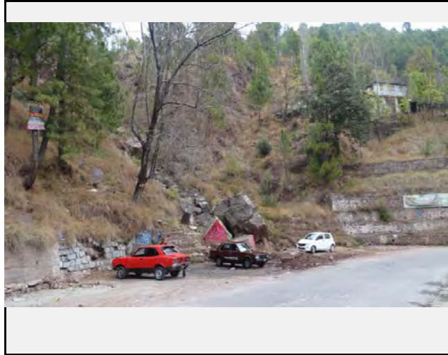
View of debris flow at start point
