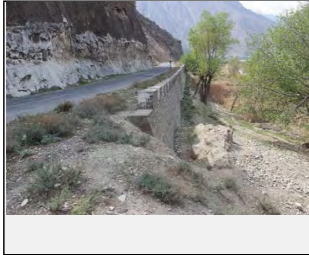
View of landslide on Valley side:
