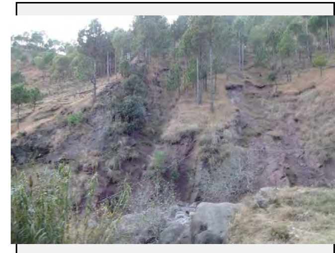
Existing countermeasures / anomalies: Several surface collapse can be observed on the west side of the slope on the mountain side.
