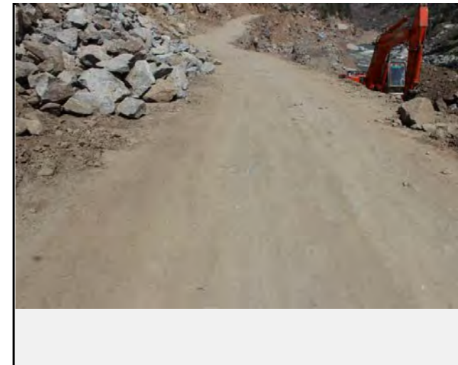
Existing countermeasures / anomalies: Retaining wall is being constructed at the toe of the debris flow
