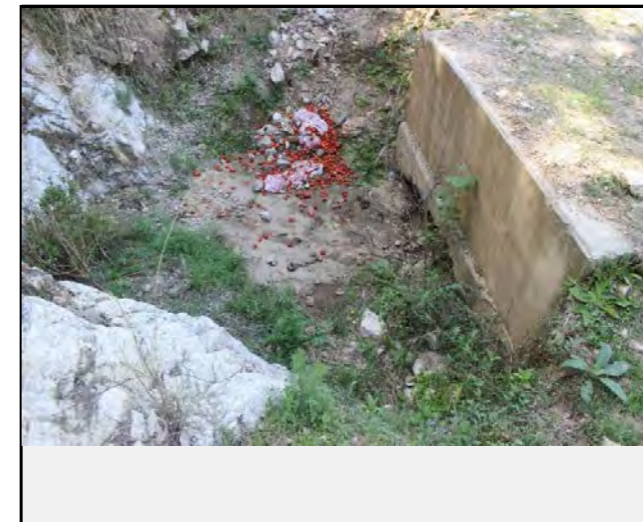
View of culvert inlet
