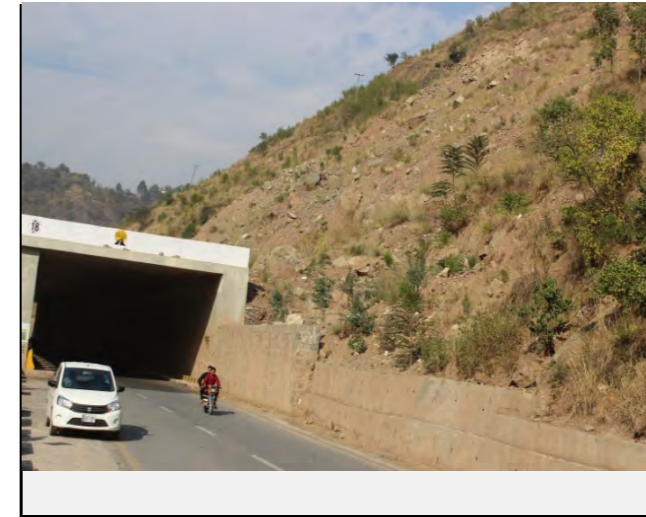
Road condition: Cut slope at the start point
