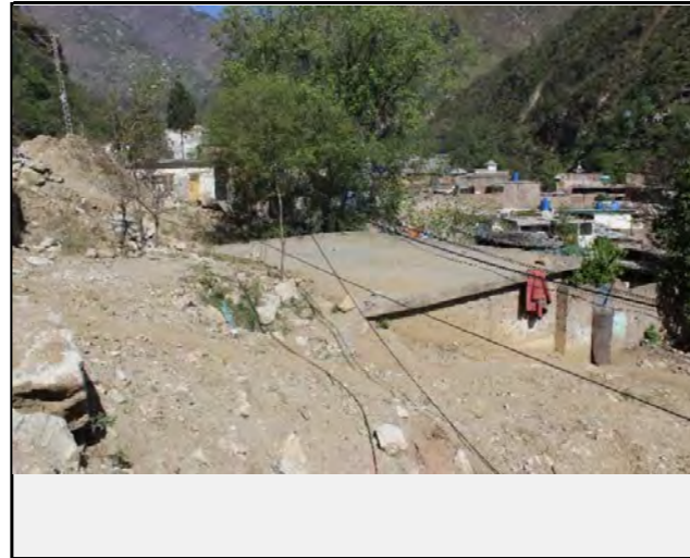
Valley side view of the debris flow
