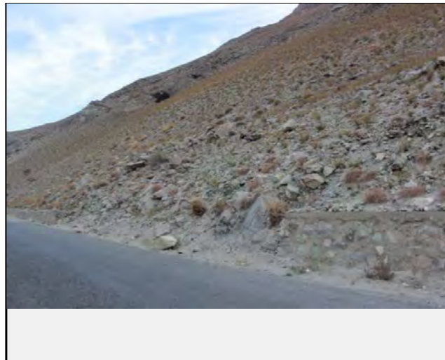
Existing countermeasures / anomalies: View of shed as counter measure
