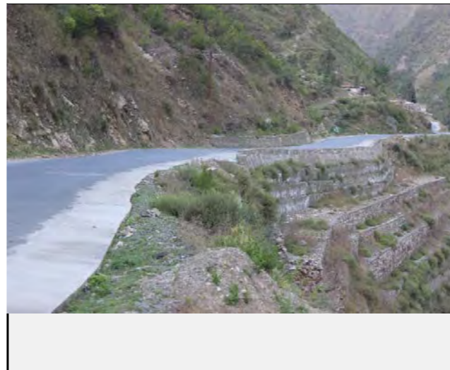
Existing countermeasures / anomalies: View of Retaining Wall as counter measure
