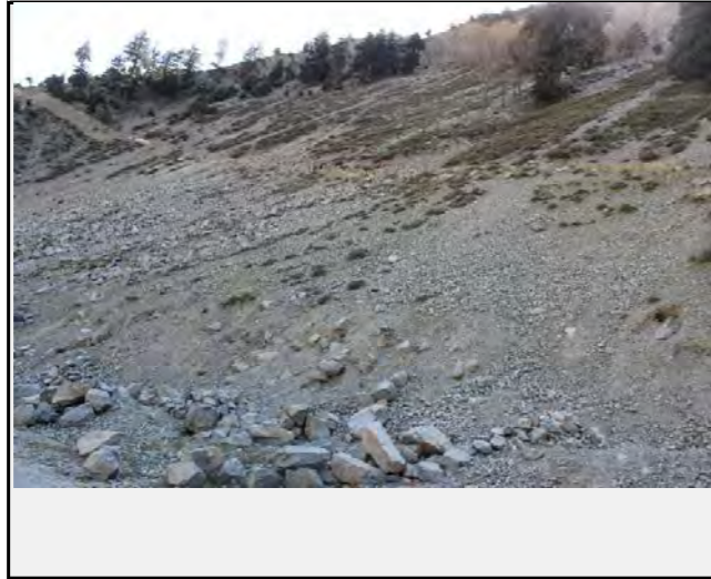
Full view of the landslide
