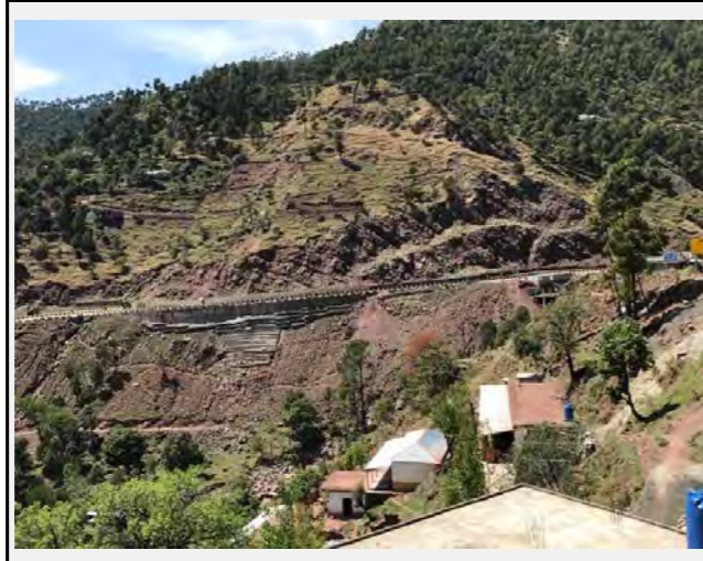
Overall view of the slope. Rock falls are expected in the mountain side and slope failure in the valley side.
