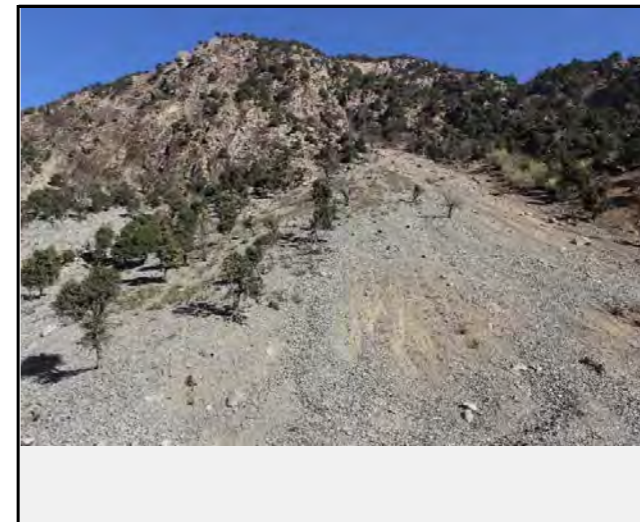
View of gully developed in the slope failure
