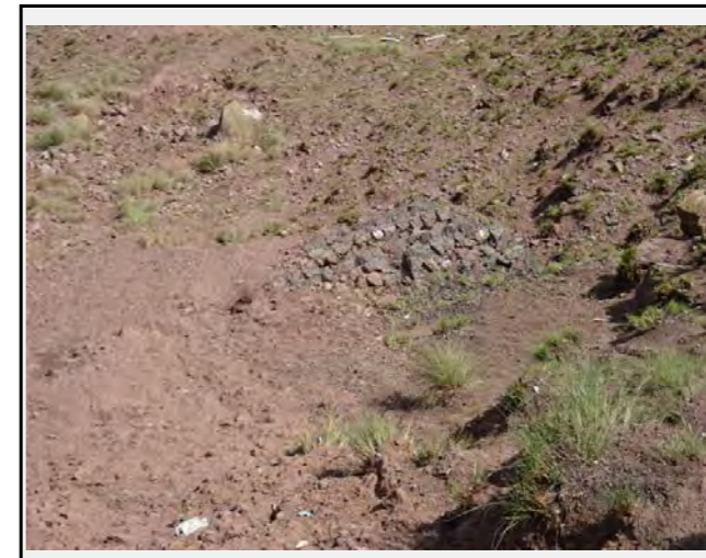
Slope failures have collapsed and damaged gabion walls constructed in the valley side as retaining walls for the embankment
