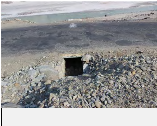
Inlet of the culvert for the debris flow
