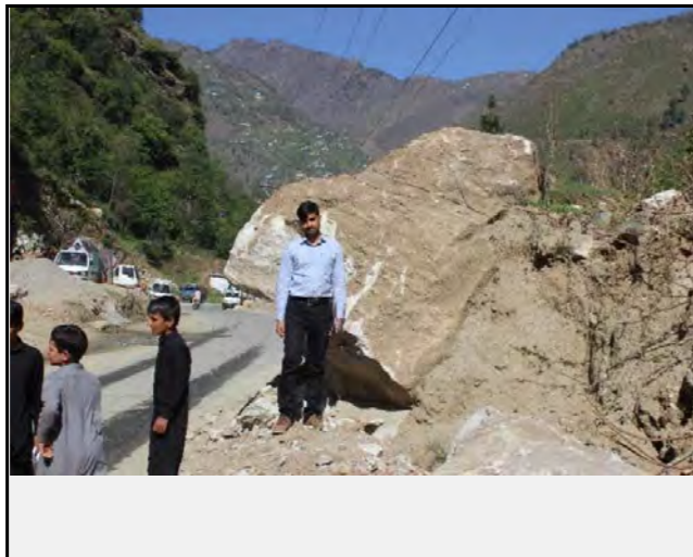
View of fallen block with the debris flow that can damage the population along the downstream.
