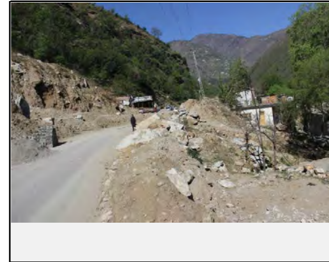
Front view of the debris flow
