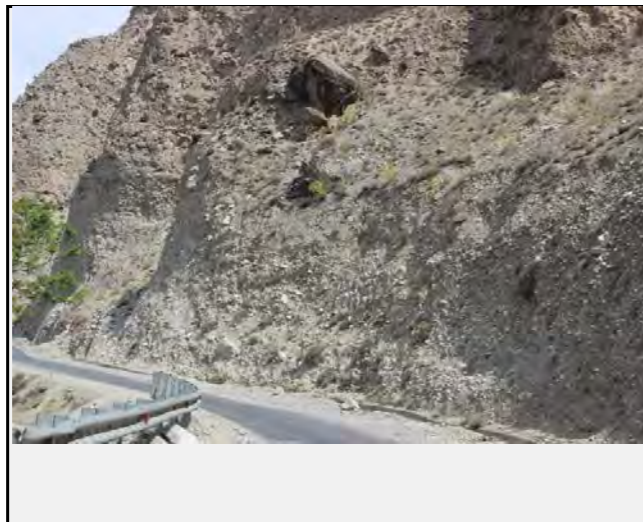
View of the slope failure at the middle point with boulder which threaten the road and traffic.
