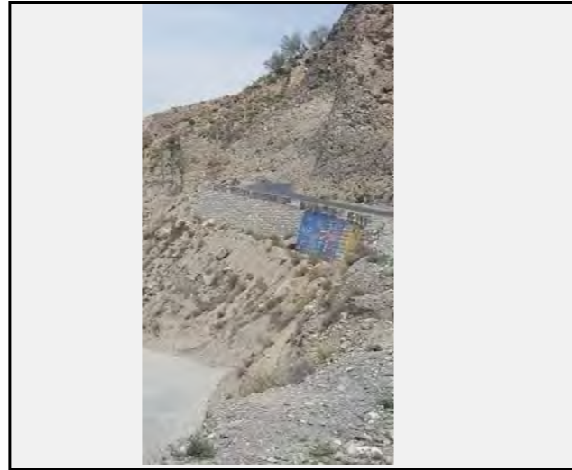
View of landslide on Valley side:
