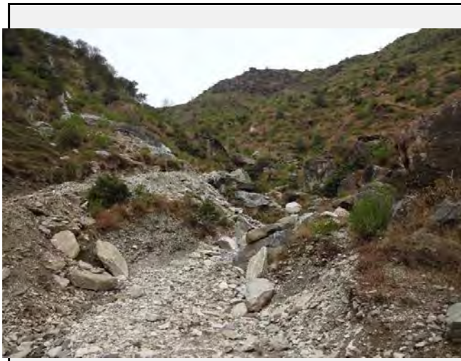
Existing anomalies: The stream is filled with debris and boulders.
