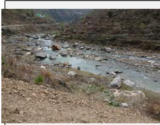
Valley side: Surface of the valley side is filled with the exavated materials from the other site.
