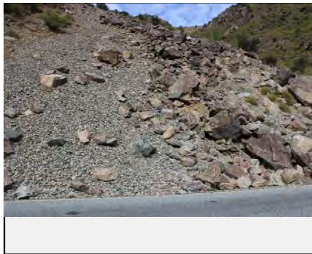
Existing countermeasures / anomalies: No counter measures
