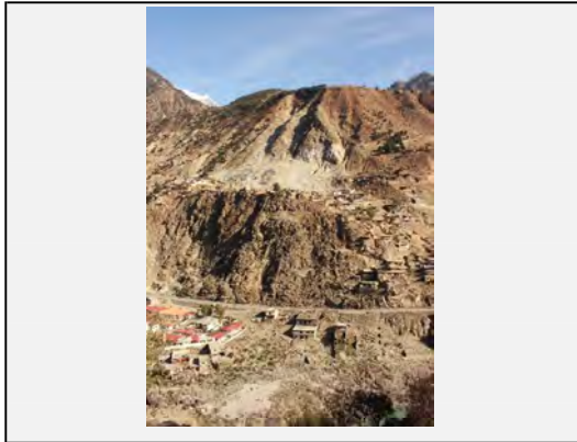
Full view of the Slope Failure/Rock Fall
