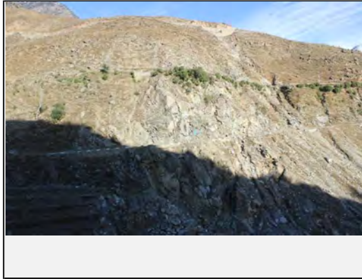
Full view of the Slope Failure
