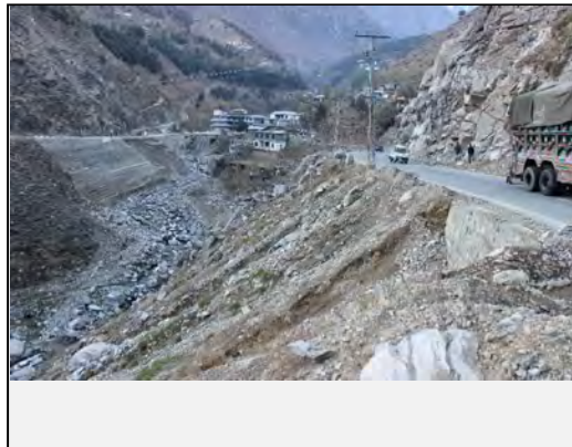
Existing countermeasures / anomalies: View of shed as counter measure
