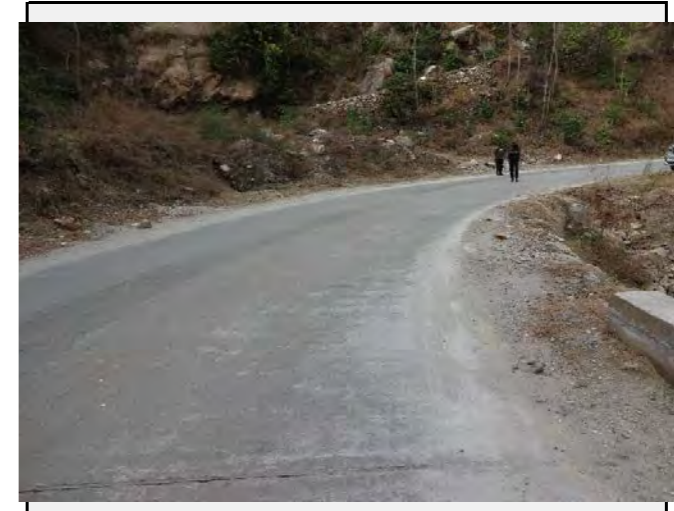
Road condition: No anomalies was observed in the causeway
