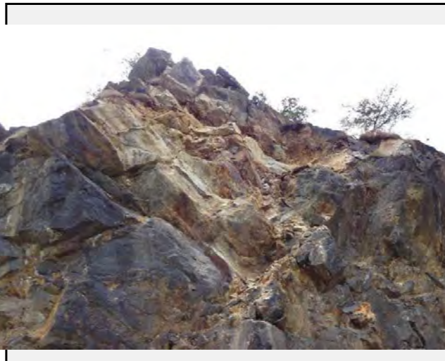
Existing anomalies: Portion of the fallen rock (from bottom)
