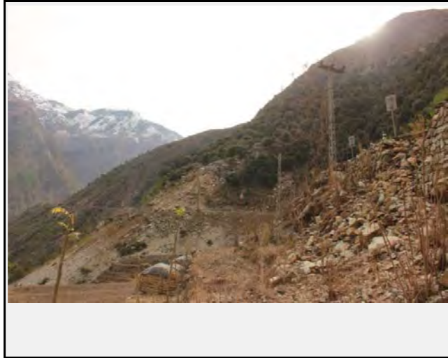
Full view of the slope failure
