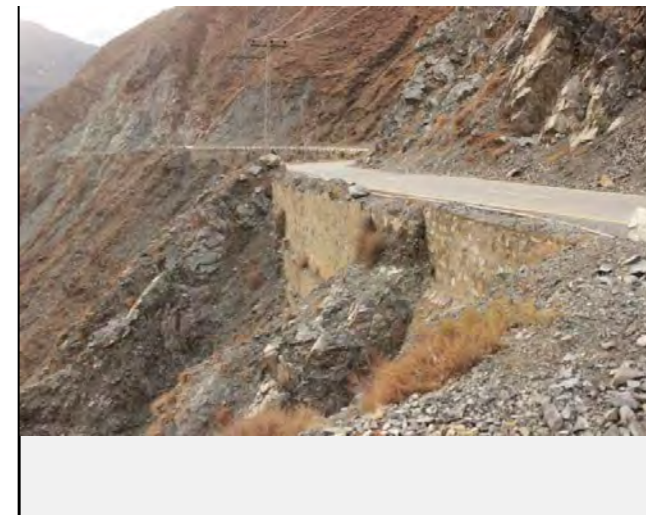
Retaining wall has been constructed to protect the road
