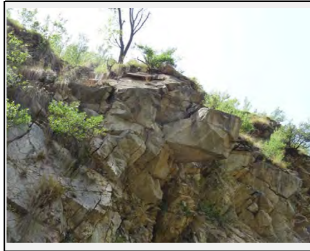
Overhangs can be observed in some spots
