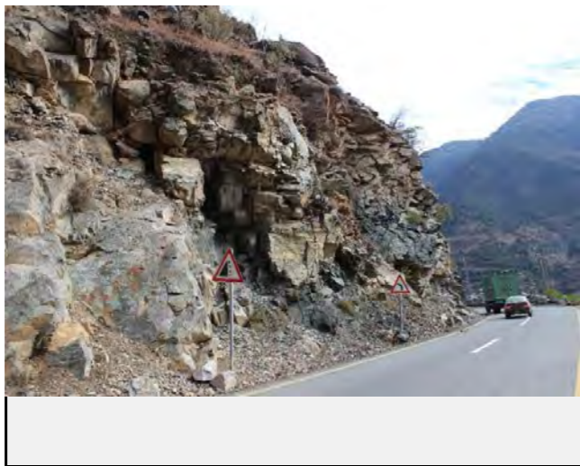
Road condition: Cut slope at the end point
