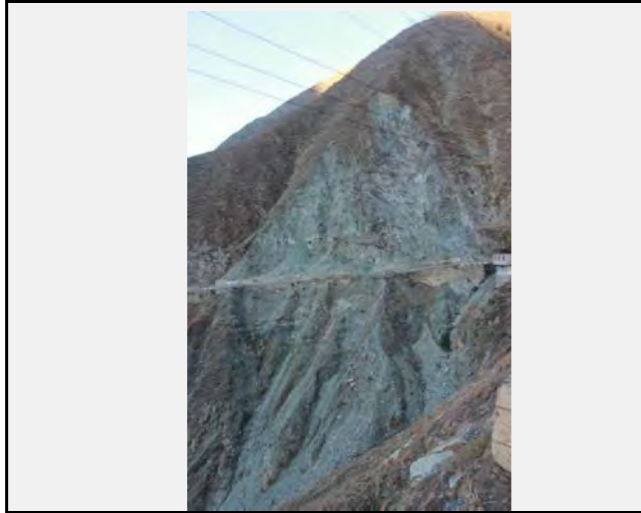
Full view of the rockfall
