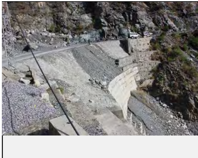
Existing countermeasures / anomalies: Sloped Retaining wall has been constructed for outflow of debris material
