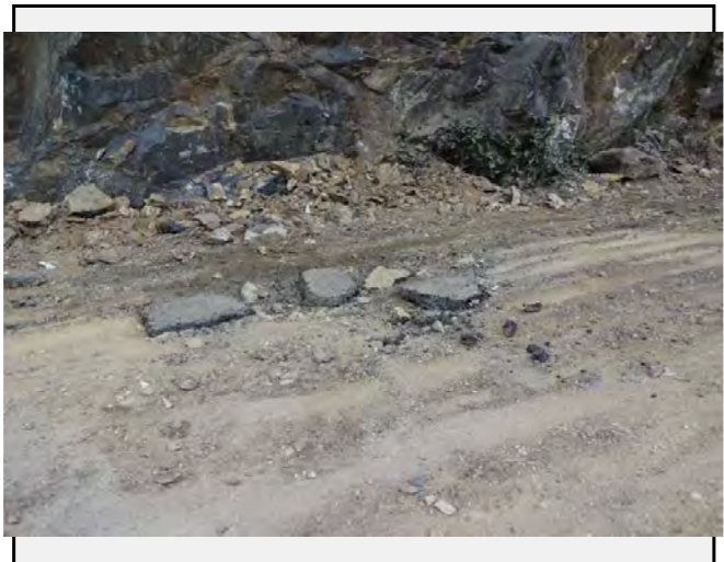
Existing anomalies: The fallen rock has damaged the road surface.
