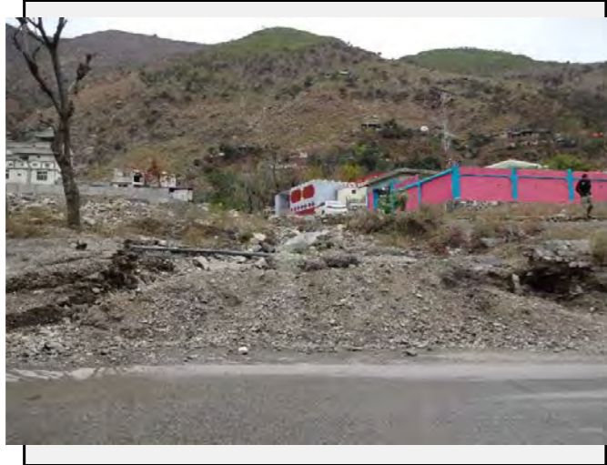
Mountain side: The exit of stream to the road is filled with the debris
