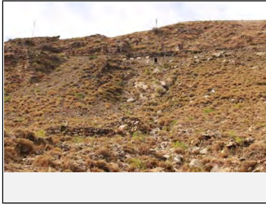
Full view of the slope failure
