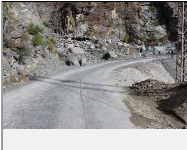
Road condition at start point
