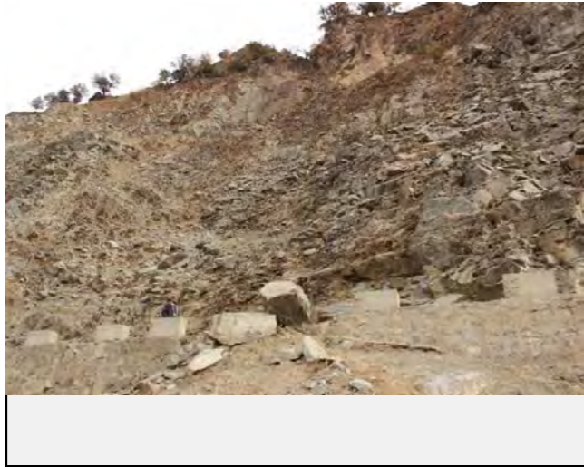
Full view of the slope failure
