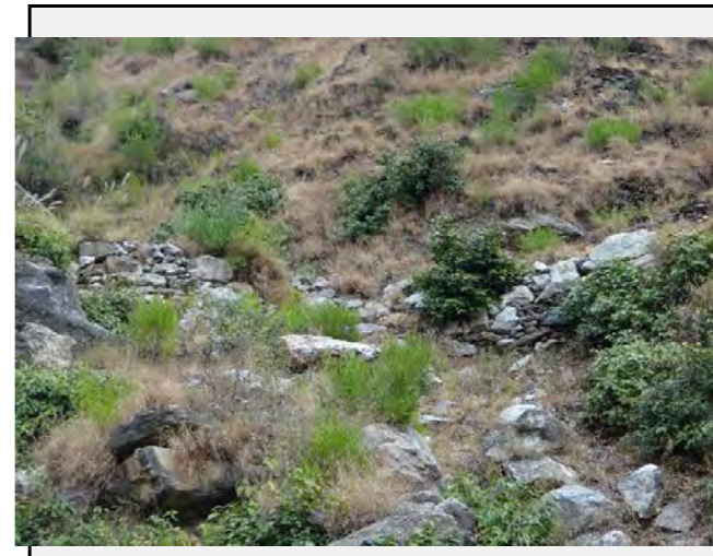
Existing countermeasures: Remains of check dam built by rocks was confirmed at the 120m from the road.
