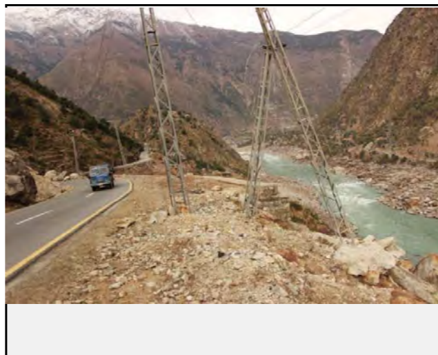
Existing countermeasures / anomalies: Retaining wall has been constructed
