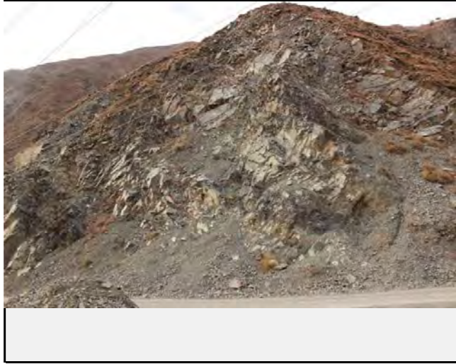
Full view of the rockfall
