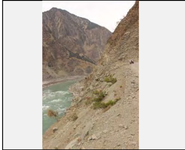
View of slope failure on Valley side:
